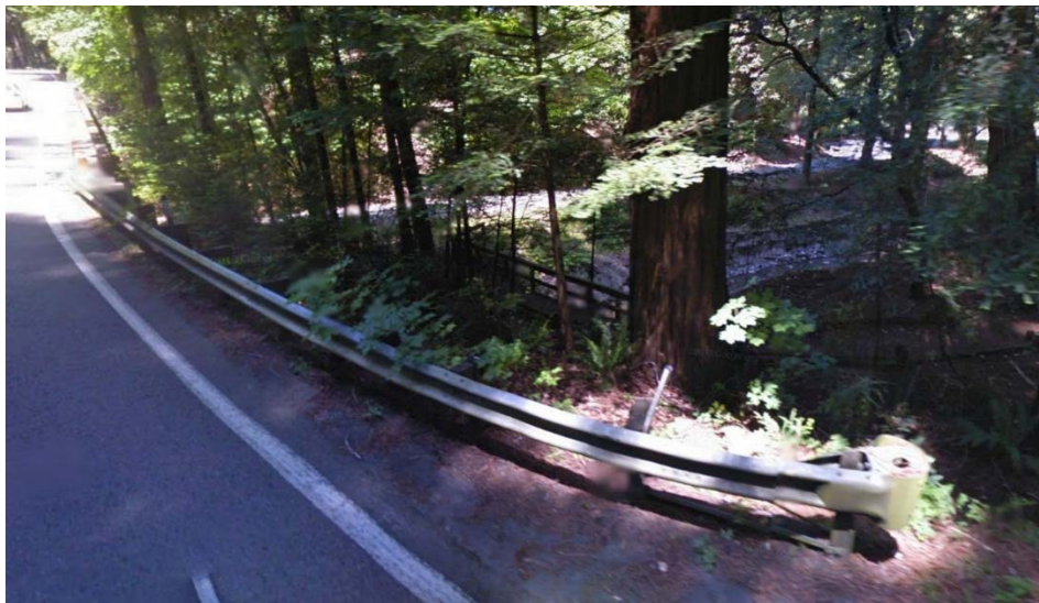
Figure 3.11 Area of Potential Riparian Disturbance (southeast of bridge)
