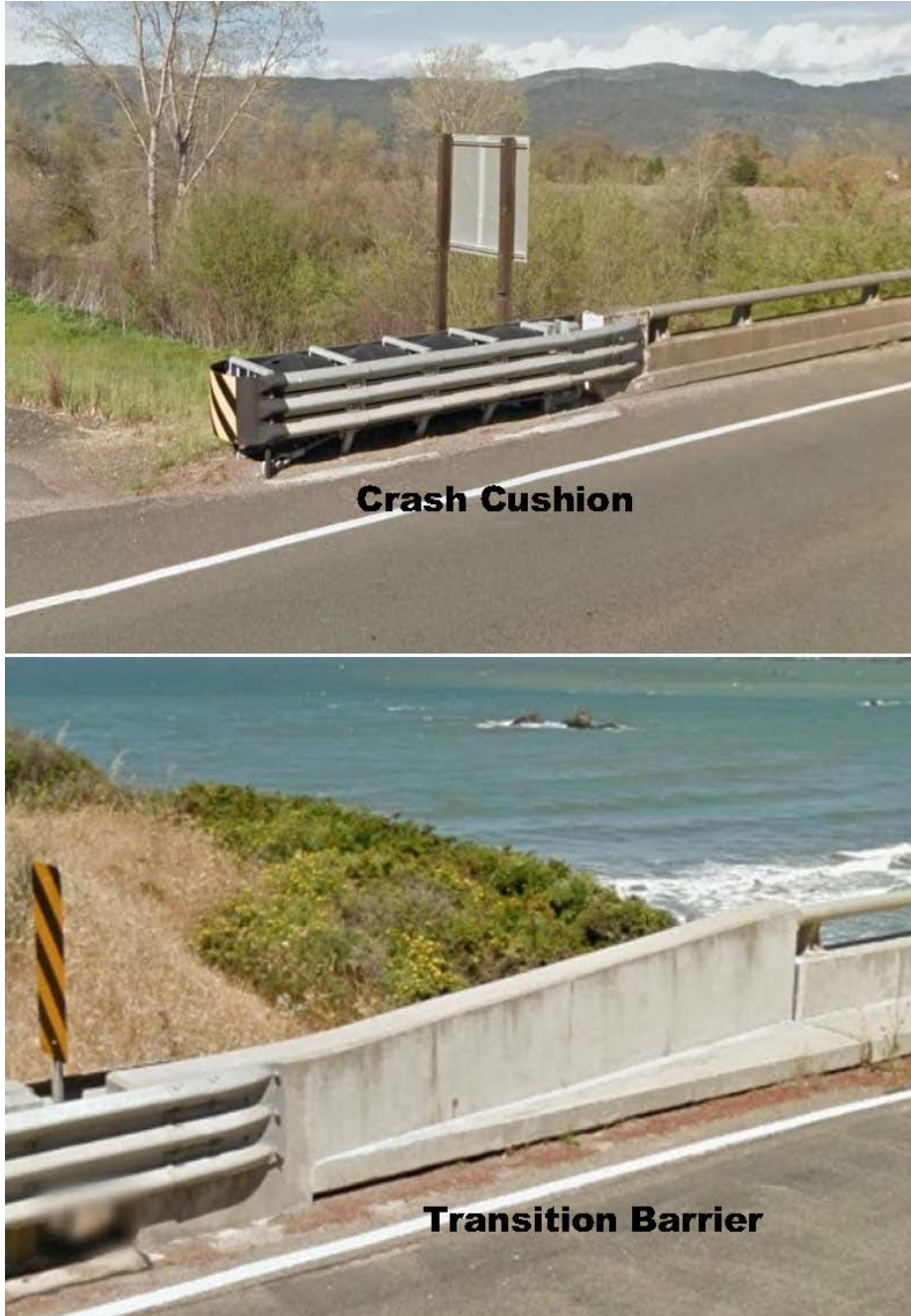
Figure 3.8 Example of Crash Cushion and Transition Barrier
