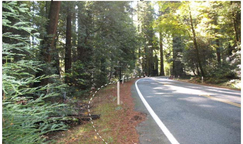
Location of sliver fill at Post Mile 1.35 to 1.40
