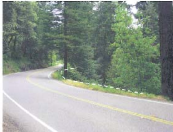
Location of retaining wall adjacent to Singing Trees Recovery Center
