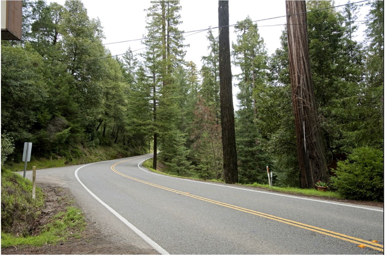
Figure 5 Before Photo at PM 2.10 outside the park looking north at where the retaining wall will be located.
