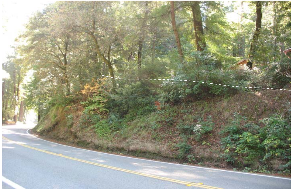
Location of cut south of Overpacks Grove Resort driveway
