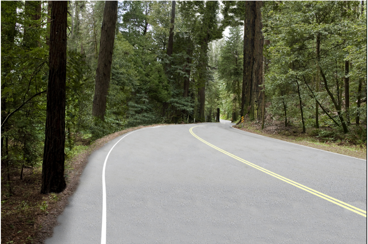
Figure 4 After Photo at PM 1.40 looking south, where greatest alignment shift of US Route 101 would occur. Centerline has shifted to the left.
