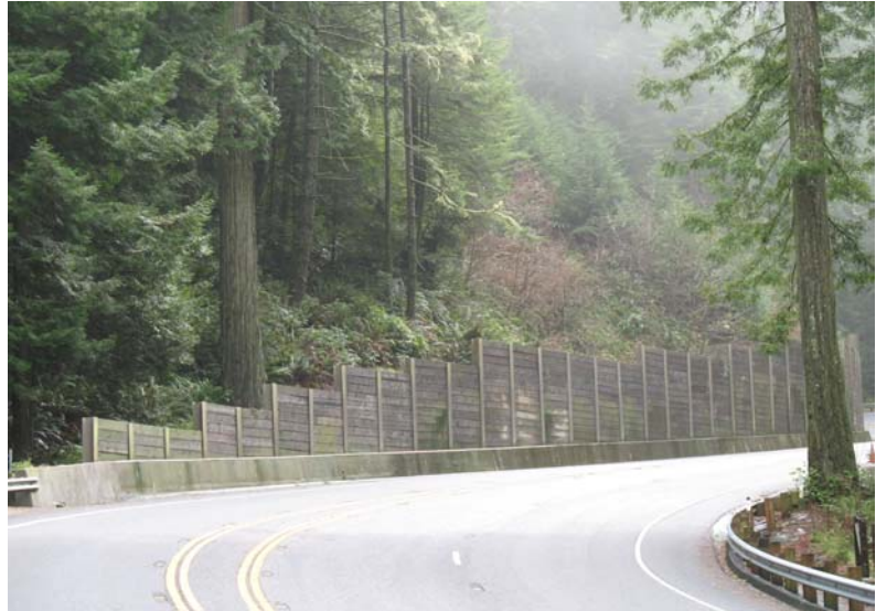
Similar type of retaining wall located in Del Norte Redwoods State Park
