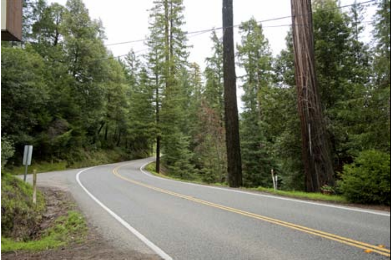
Figure 5 Before Photo at PM 2.10 outside the park looking north at where the retaining wall will be located.
