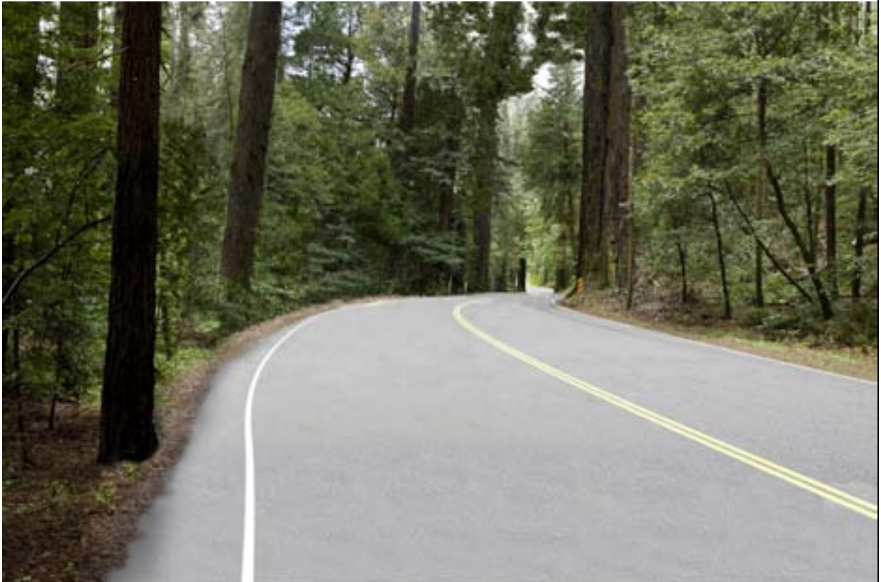
Figure 4 After Photo at PM 1.40 looking south, where greatest alignment shift of US Route 101 would occur. Centerline has shifted to the left.
