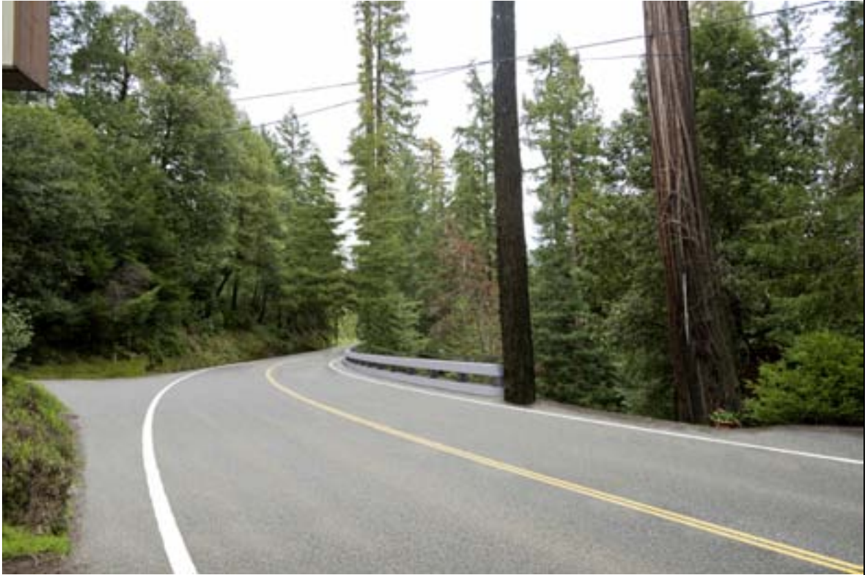
Figure 6 After Photo at PM 2.10 outside the park looking north at the barrier for the retaining wall.
