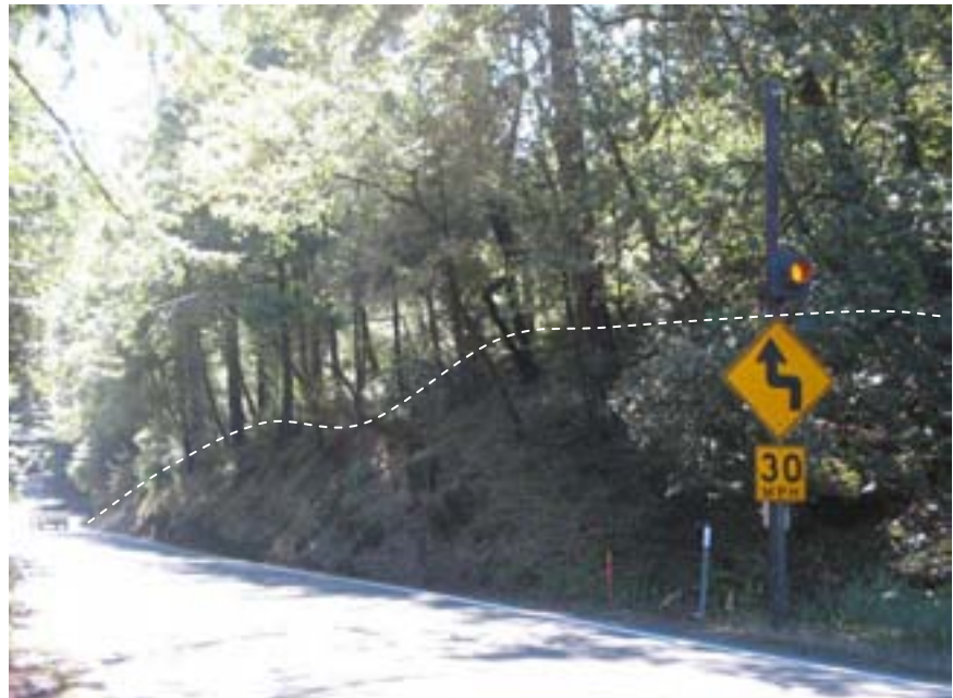
Location of retaining wall north of Overpacks Grove Resort driveway
