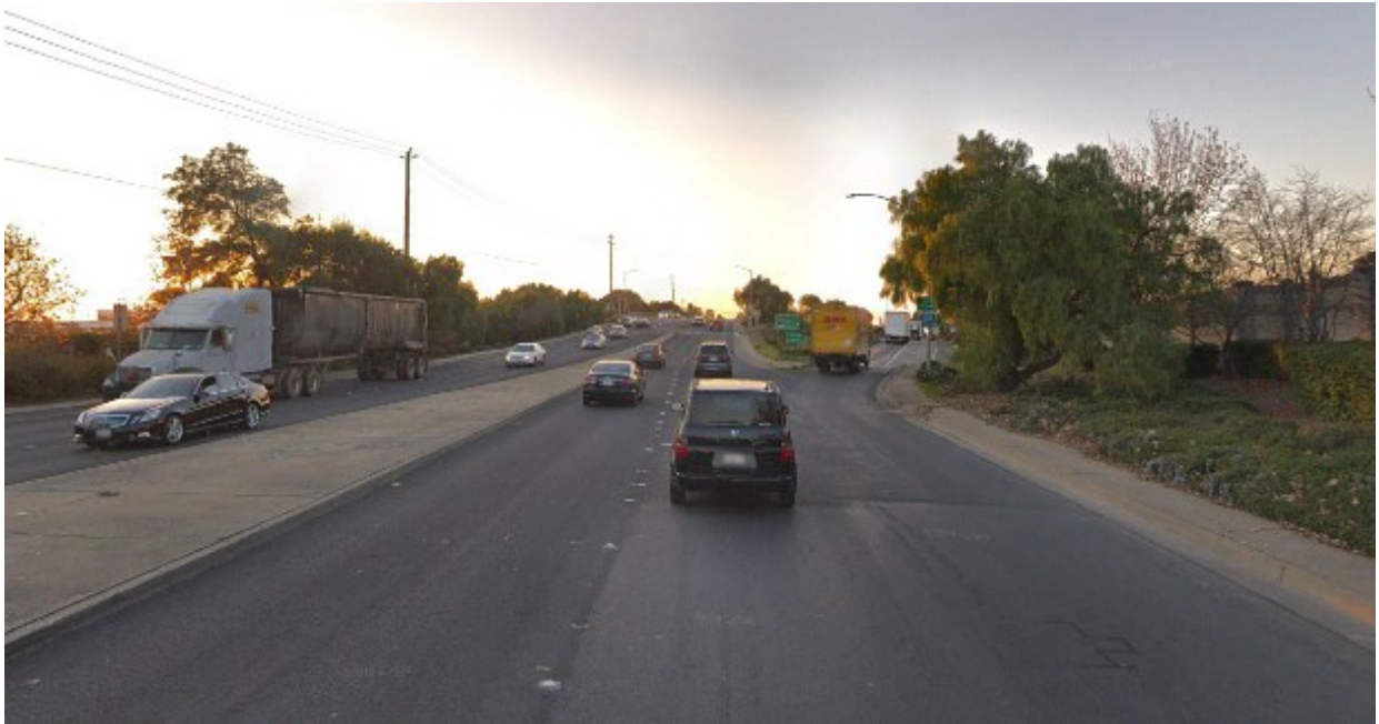
Figure 2.1-9 Viewpoint 5: Industrial Parkway West (Existing Condition)
