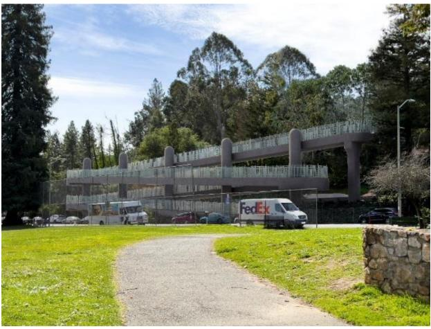
Figure 2-4. Alternative 2. Proposed pedestrian overcrossing and switchback ramp in green space between SR-13 and Moraga Ave. as viewed from Montclair Park trail. View southwest.
