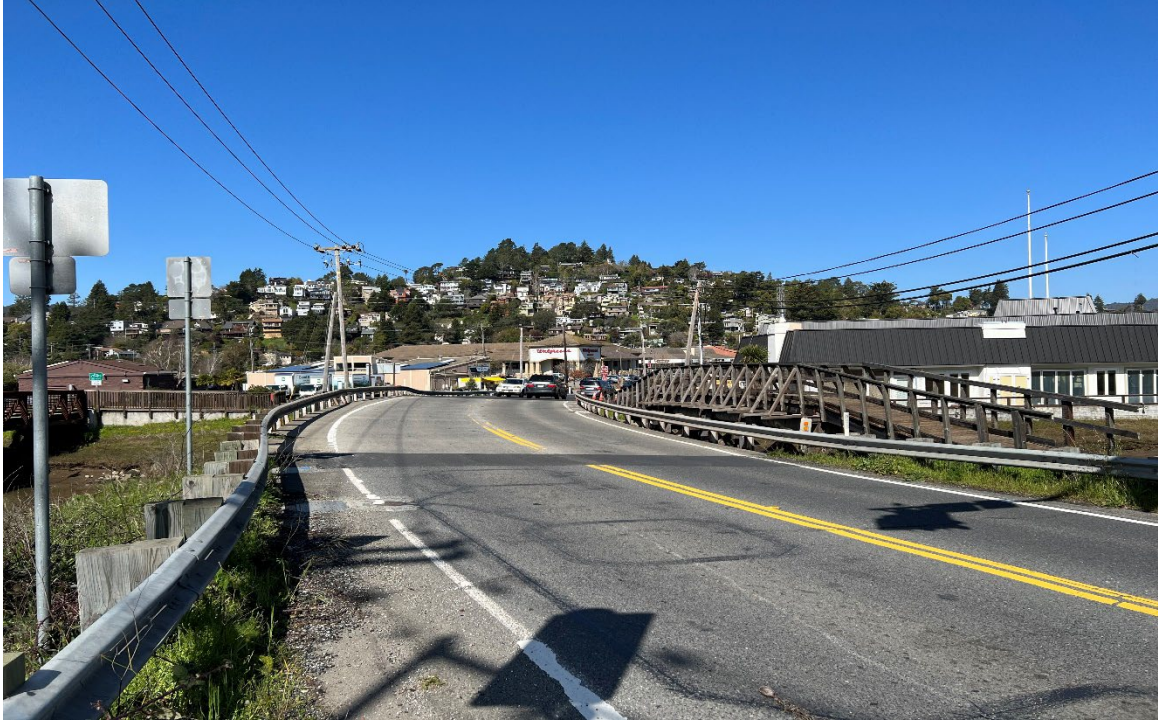
Figure 3.3.1-1. Coyote Creek Bridge Existing Conditions Northbound View
