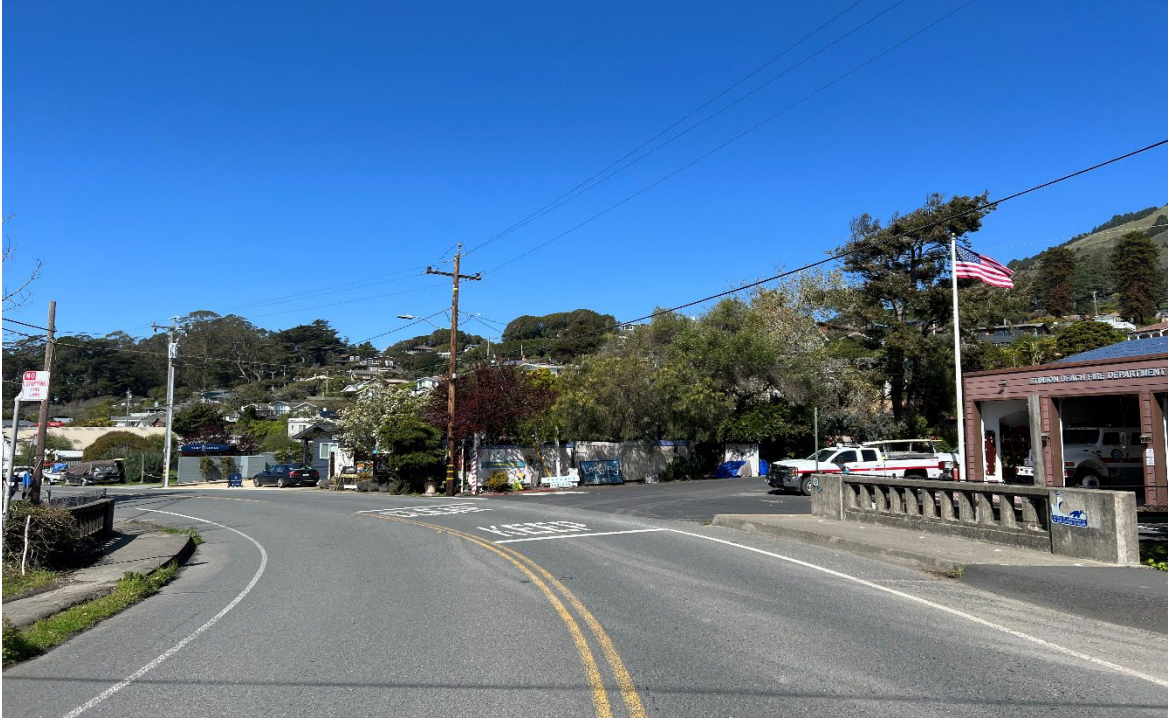
Figure 3.3.1-3. Eskoot Creek Bridge Existing Conditions Northbound View
