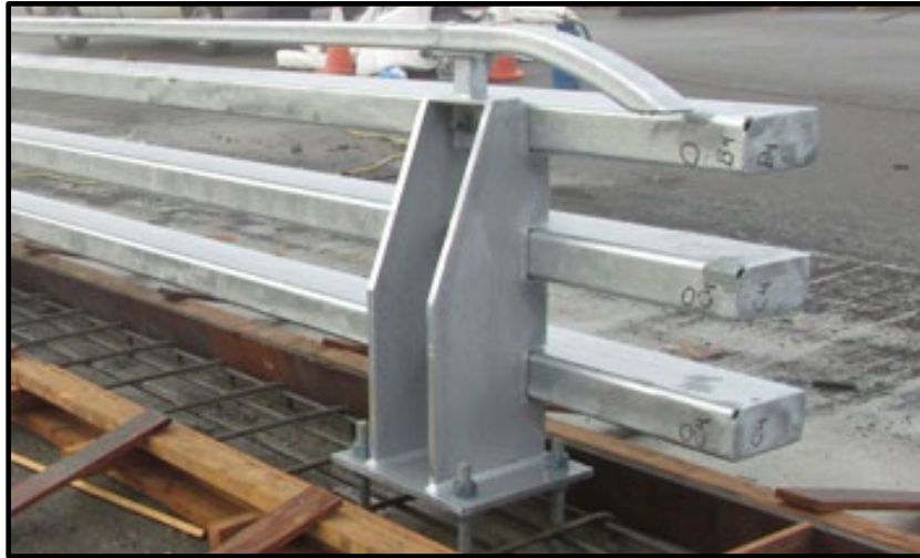
Figure 2-1 Example of a CA ST-75 Bridge Rail
