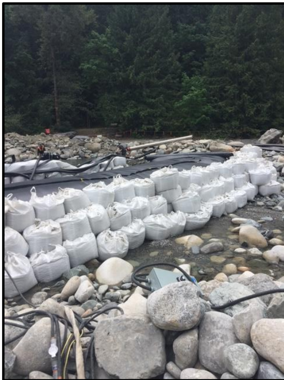
Figure 2-2 Examples of a Temporary Creek Diversion System
