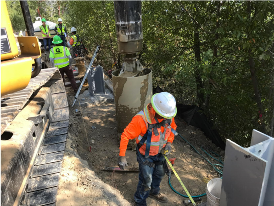
Figure 1-6 Examples of Barrier Installations (Page 2 of 2)
