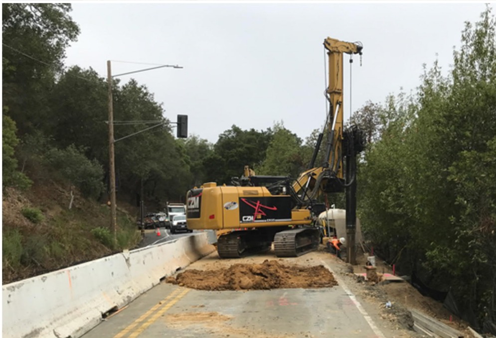
Figure 1-6 Examples of Barrier Installations (Page 1 of 2)
