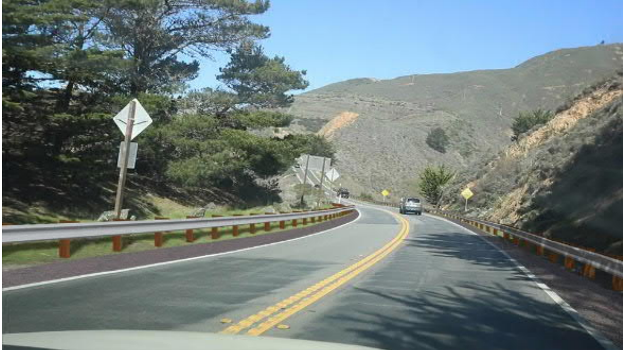
Build Alternative 2 with 5-foot shoulders and MGS
