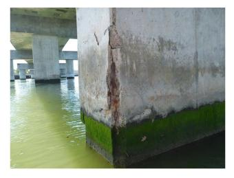
Photos from Bridge Inspection Report: Existing Column Conditions
