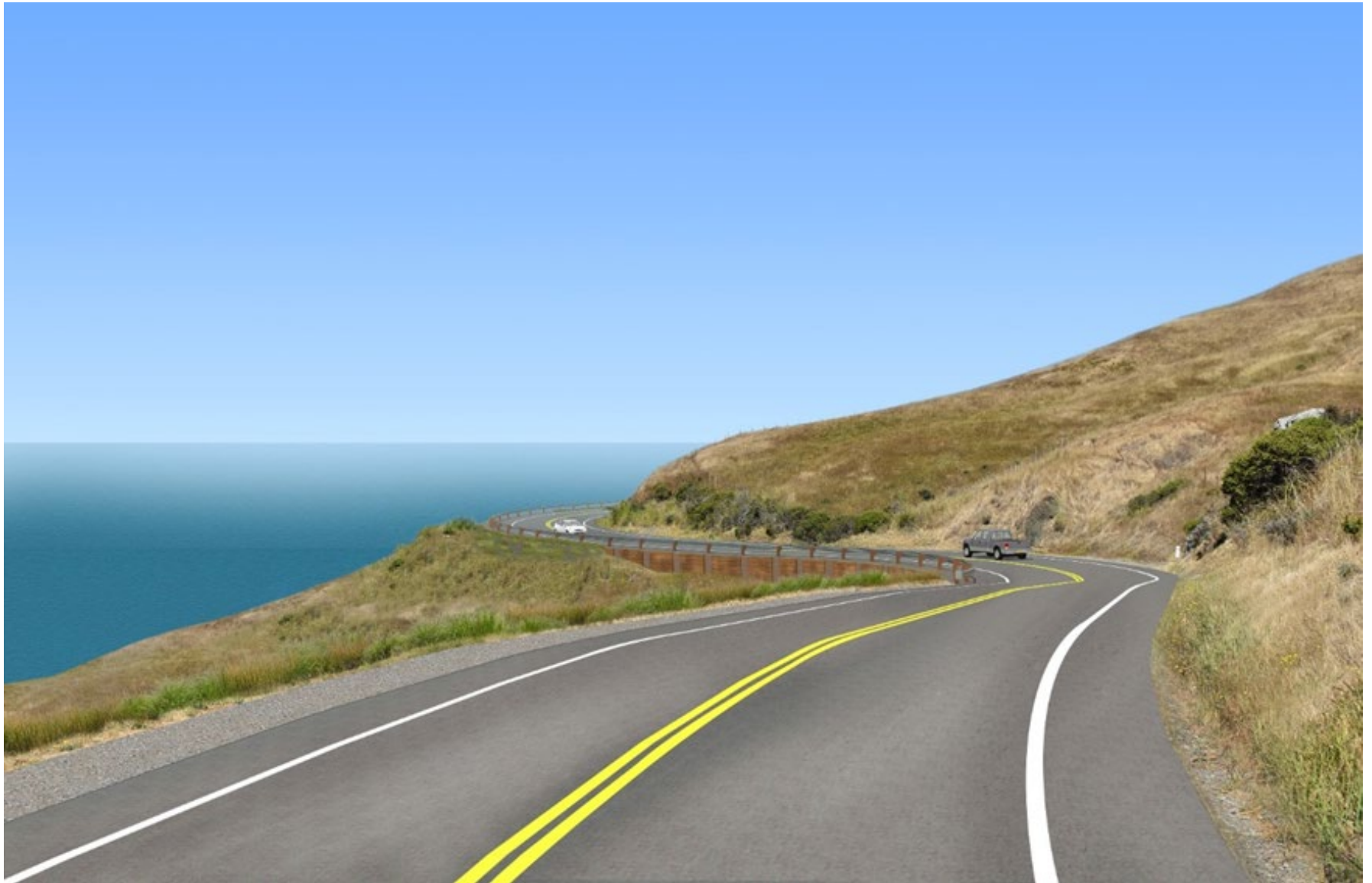
Figure 3-2 Facing Northbound – Wall Mostly Buried
