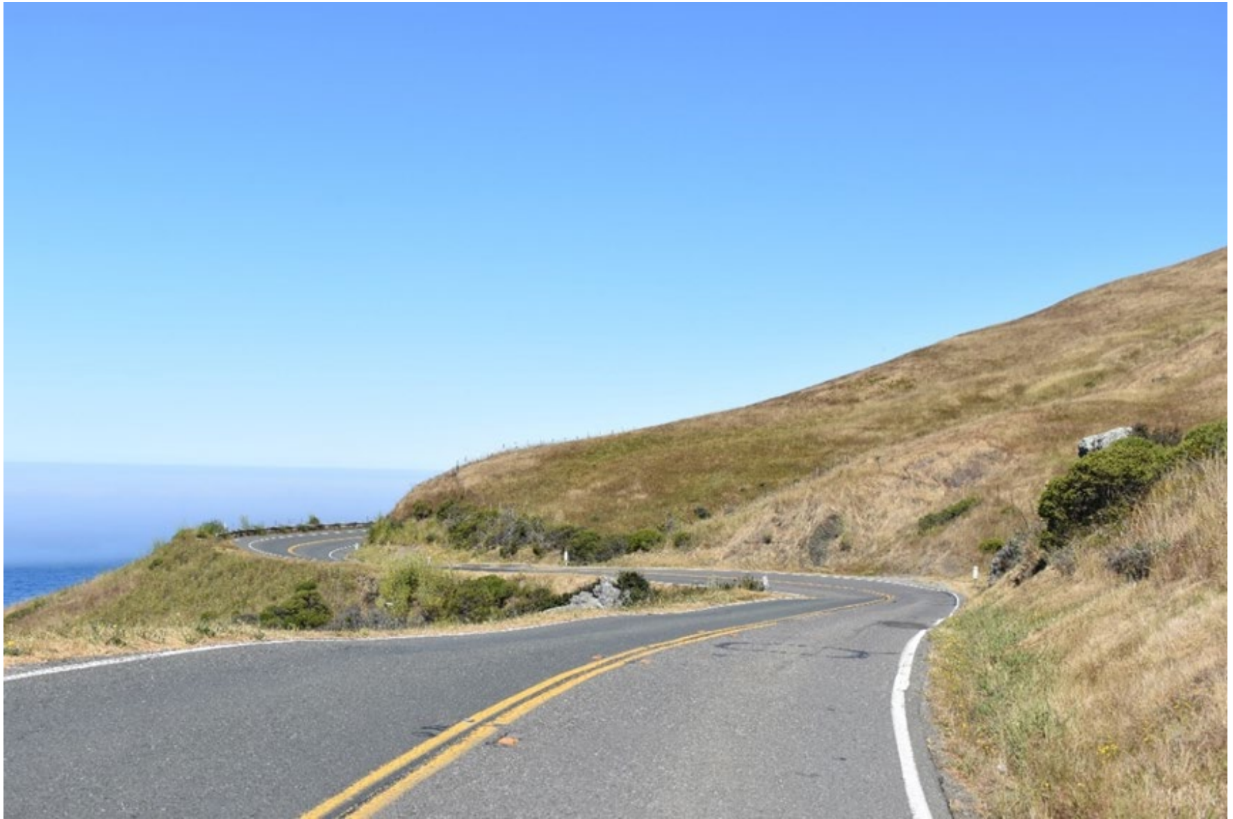
Figure 3-1 Facing Northbound – Existing Condition
