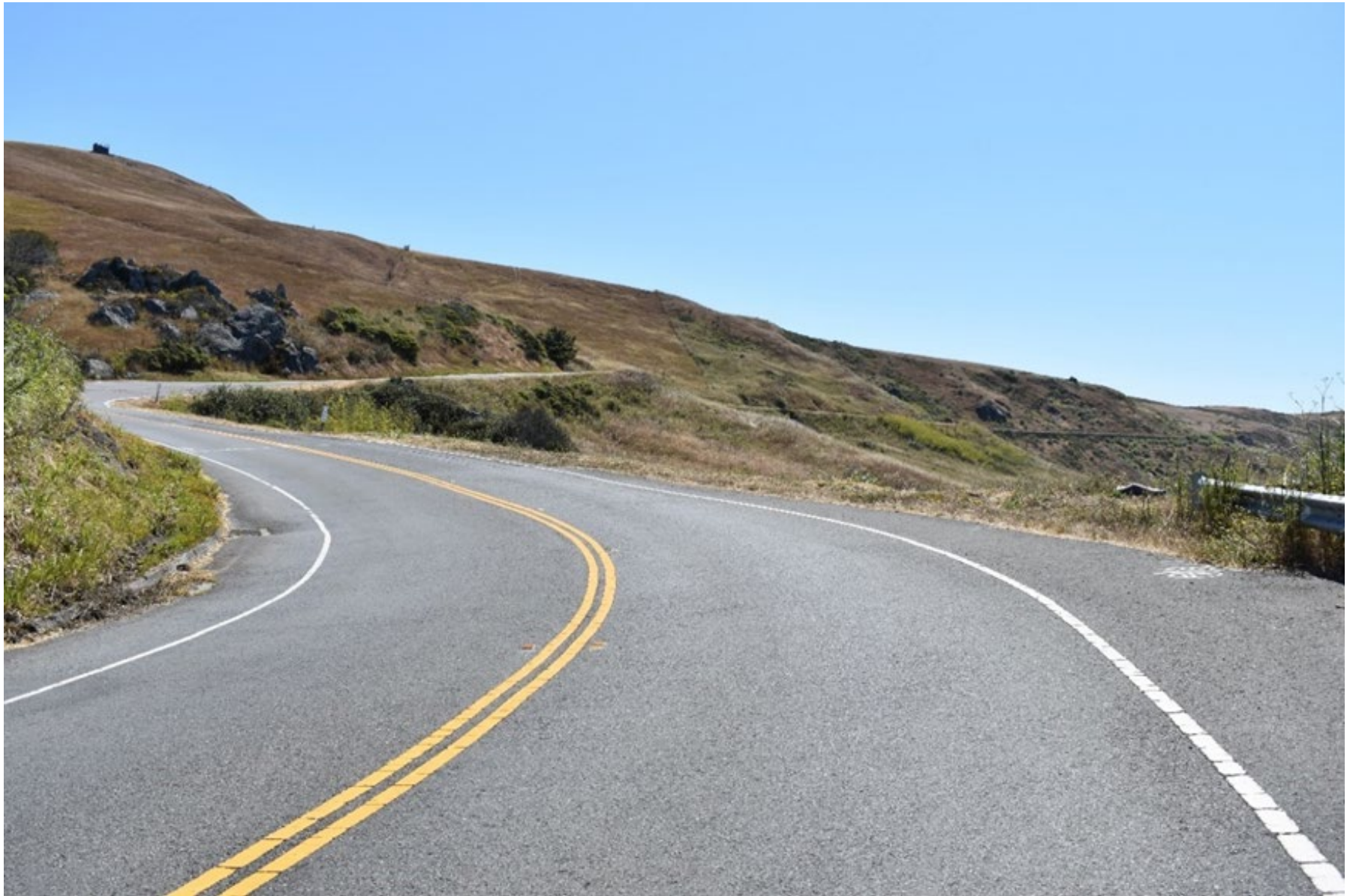
Figure 3-4 Facing Southbound – Existing Condition
