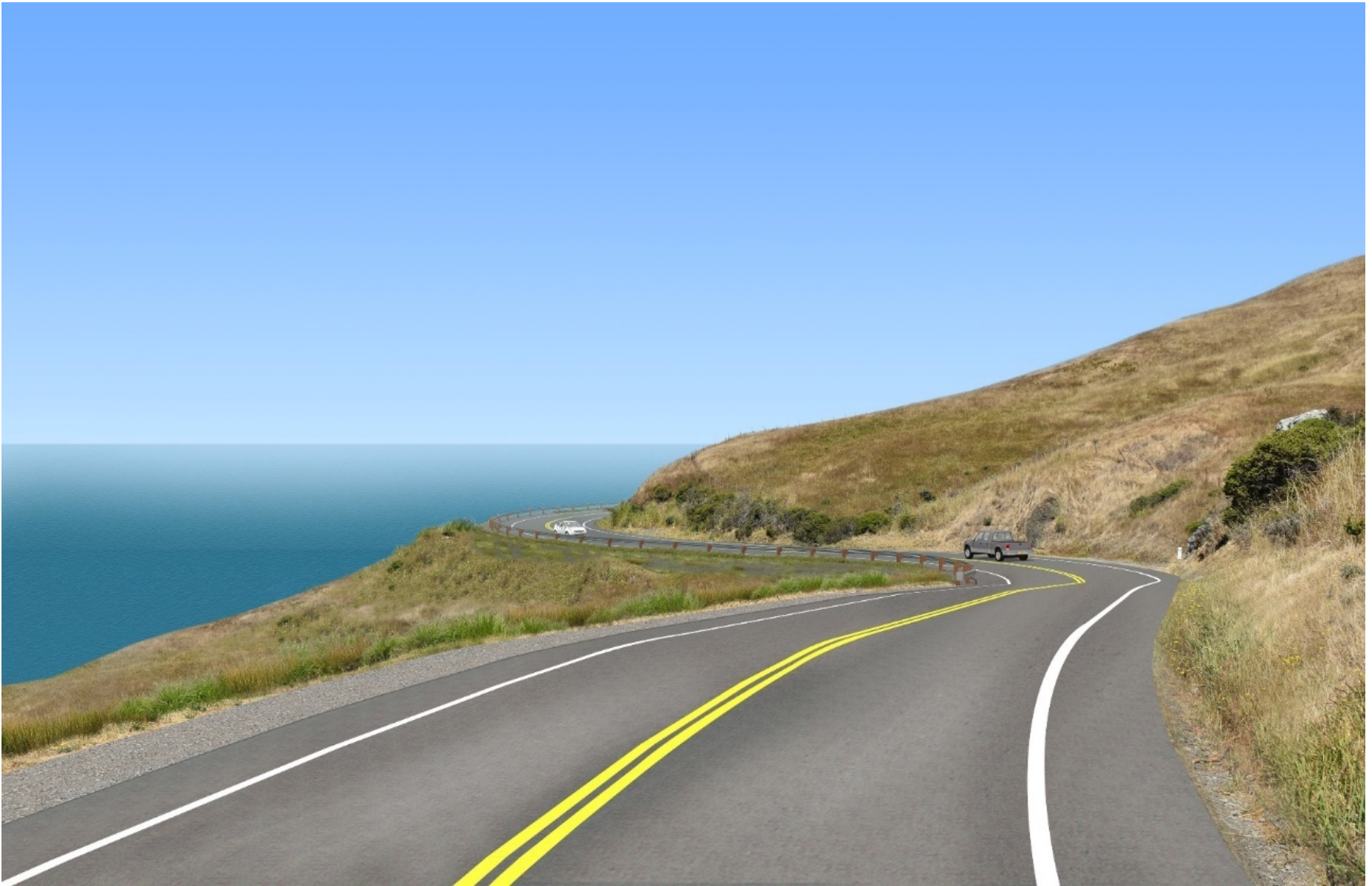
Figure 3-3 Facing Northbound – Wall Fully Buried
