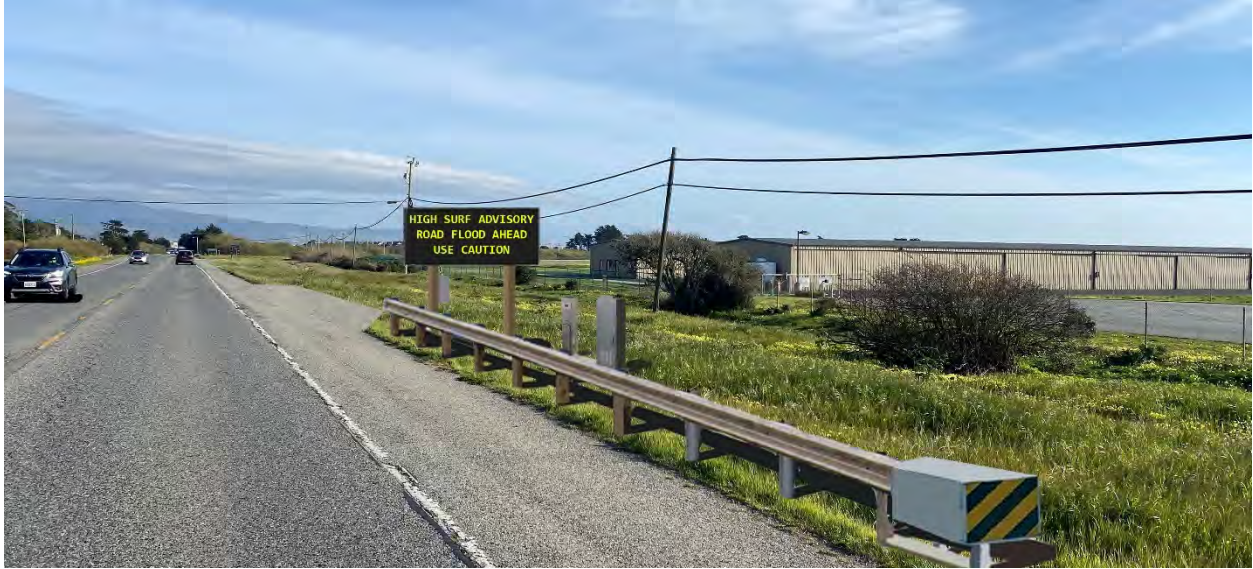
Figure 1-15 Visual Simulation of VMS (shown with message displayed) and MGS at Location 5
