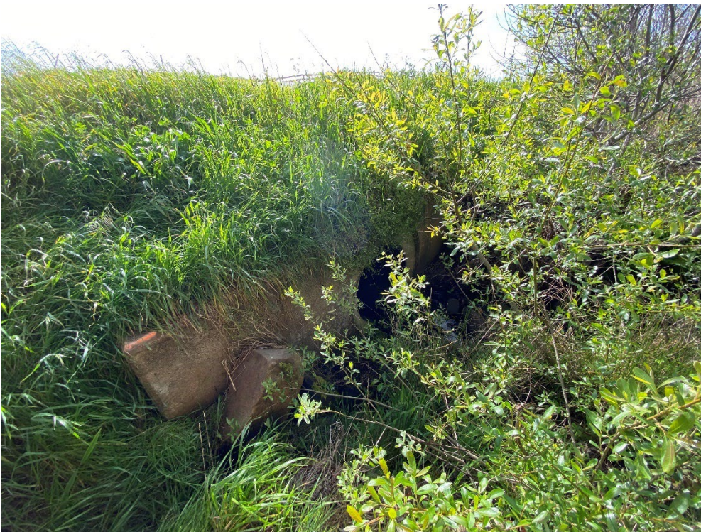
Photo 2. Culvert Inlet and Headwall
