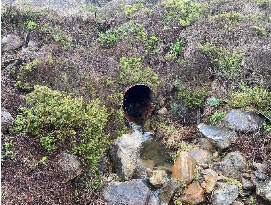
Photo 1. Existing Culvert Condition at the Downstream End
