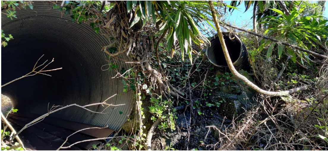
Photo 3. Culvert Outlets at Locations 2 and 3 – PM 21.84, Looking East
