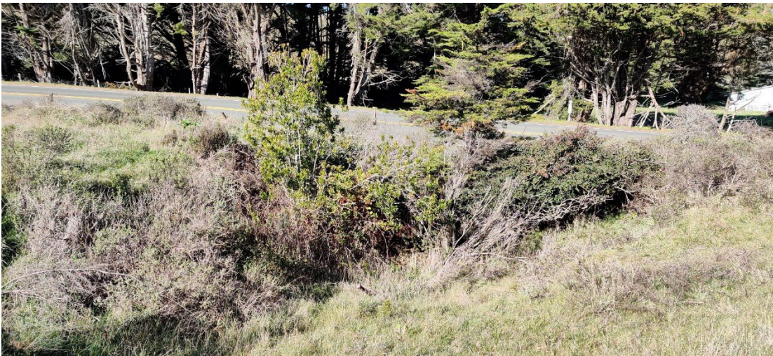
Photo 2. Culvert Location 1 Inlet – PM 19.25, Looking North
