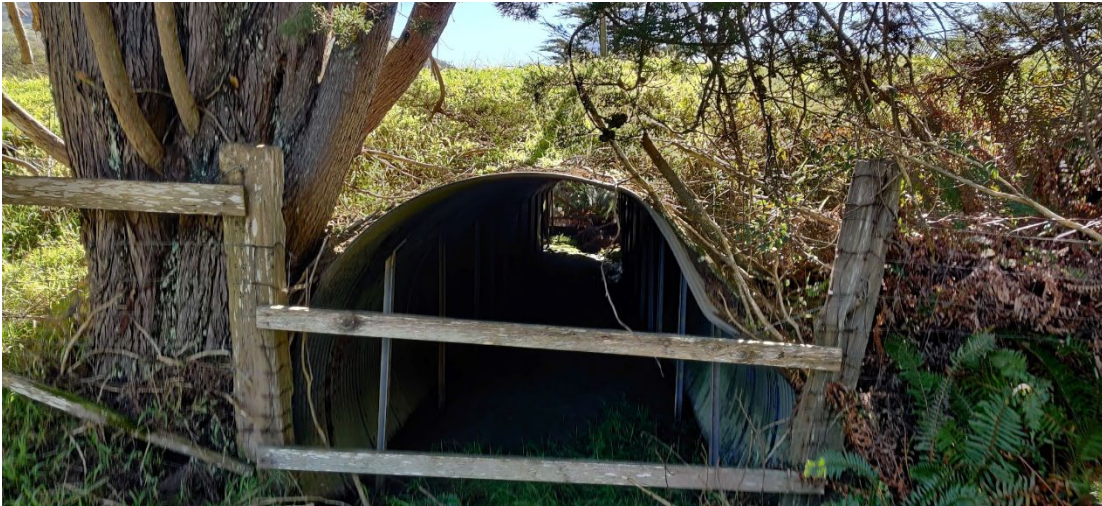
Photo 1. Culvert Location 1 Outlet – PM 19.25, Looking South
