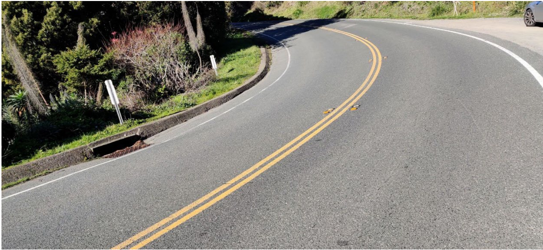
Photo 5. View of drainage inlet at Culvert Location 2 – PM 21.84, Looking West
