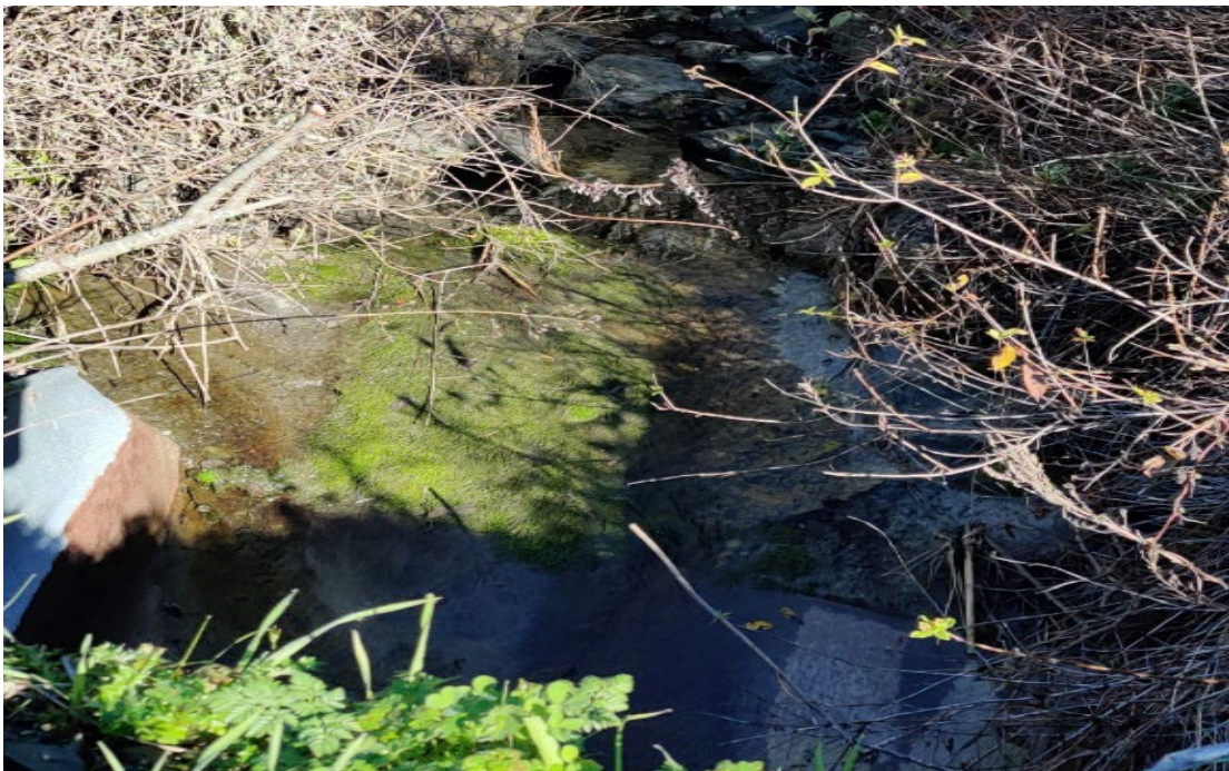
Photo 4. Culvert Location 3 Inlet – PM 21.84, Looking Northeast
