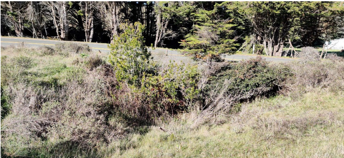
Photo 2. Culvert Location 1 Inlet – PM 19.25, Looking North
