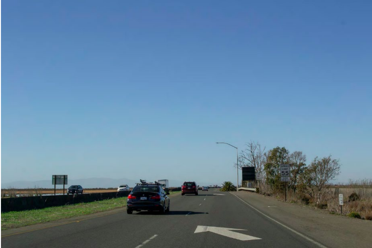
Figure 2-1 Existing Conditions from KV-1
