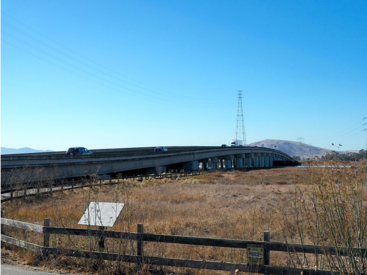
Figure 2-12 Existing Condition KV-4
