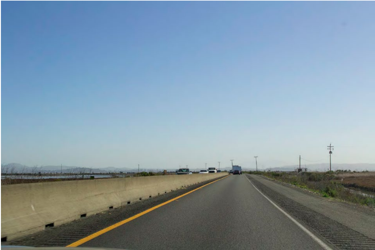
Figure 2-8 Existing Condition KV-3
