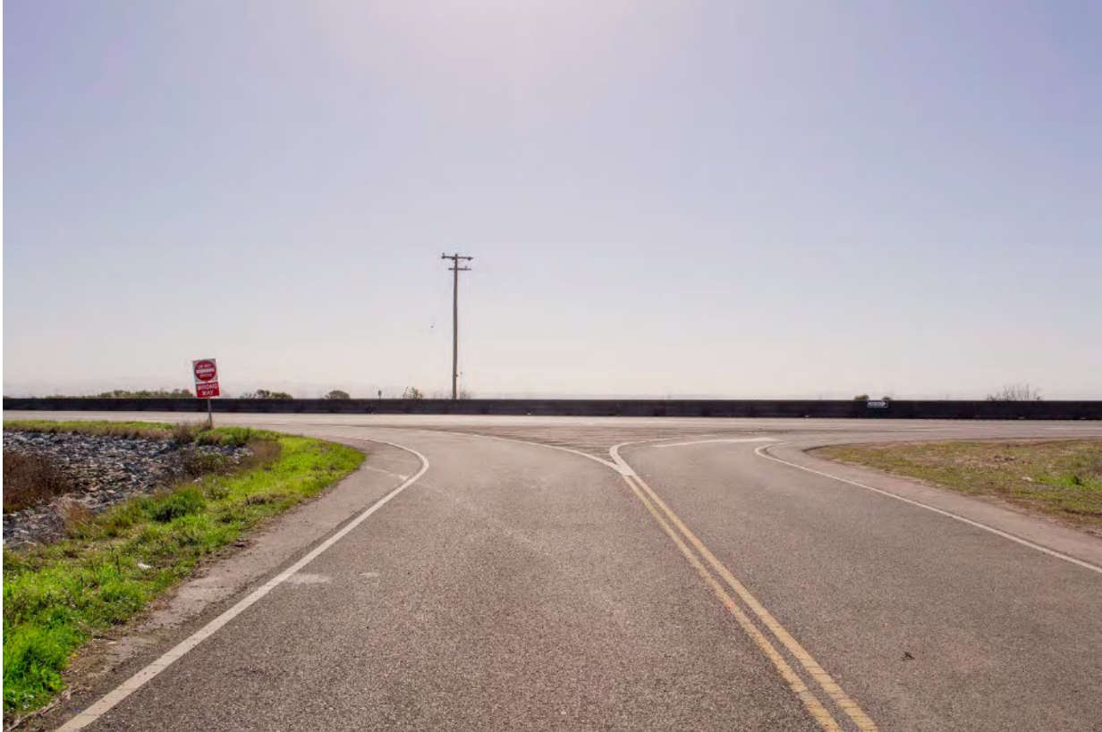
Figure 2-5 Existing Condition at KV-2
