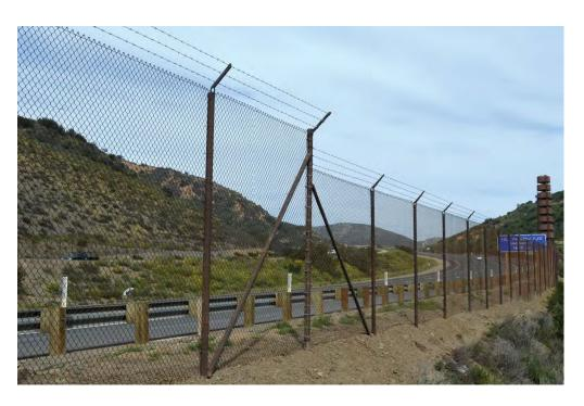
Figure 1.4-5: Example of wildlife fencing along SR 241 in Orange County, CA (McFall et al. 2015)
