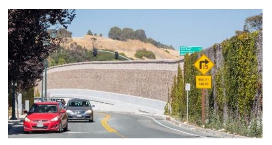
Figure 1.4-7: Example of a masonry sound wall on top of a concrete barrier, El Portal Drive, San Pablo, CA (AECOM 2020). The height, color, and materials used for this project may differ
