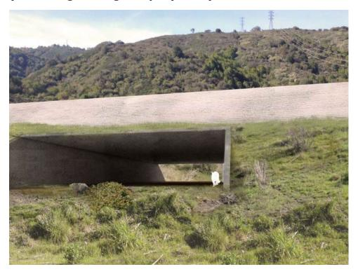
Figure 1.4-4: Simulated view of a concrete slab unit bridge, facing west toward the wildlife undercrossing and Trout Creek, below northbound SR 17 (Midpen 2019)
