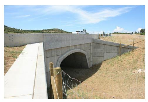
Figure 1.4-3: Example of a precast arch wildlife undercrossing with wingwalls and directional fencing, at U.S. Highway 160 in southern Colorado (Muller Engineering Company 2022)
