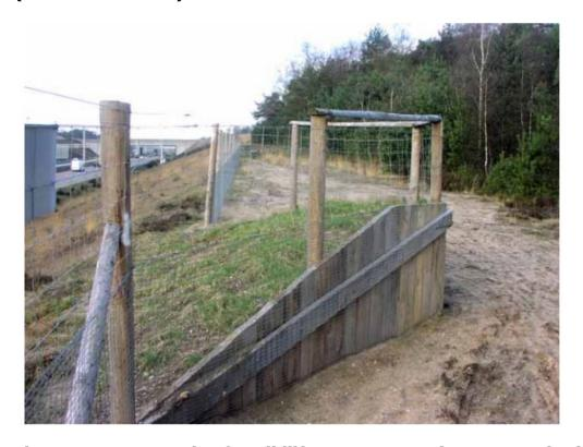
Figure 1.4-6: Example of a wildlife escape ramp (FHWA 2011). The height, color, and materials used for this project may differ
