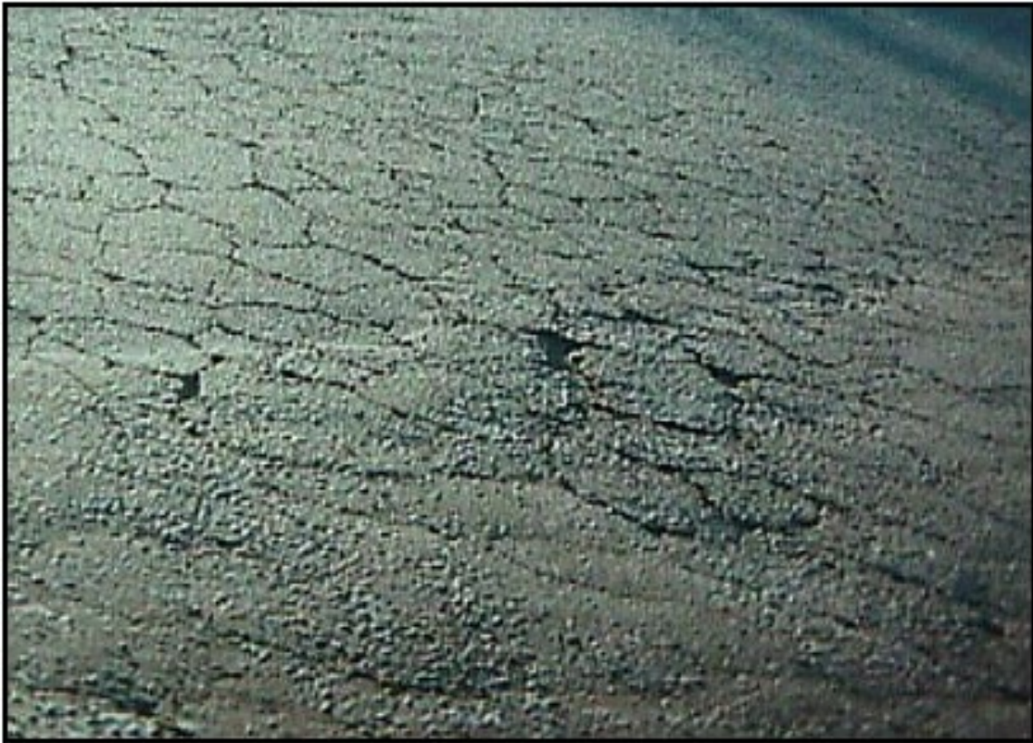
Figure 1.3.2-1: Roadway Cracking
