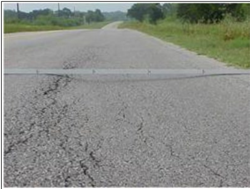
Figure 1.3.2-3: Roadway Rutting
