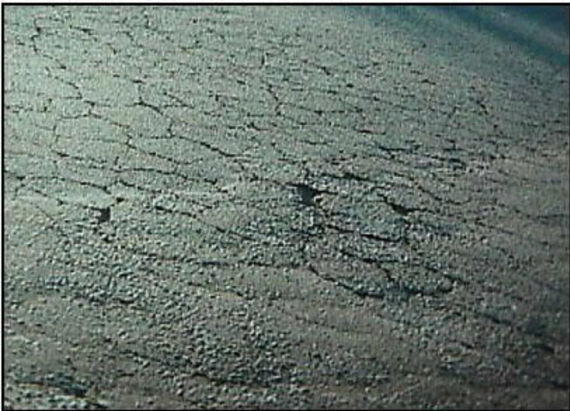
Figure 1.3.2-1: Roadway Cracking
