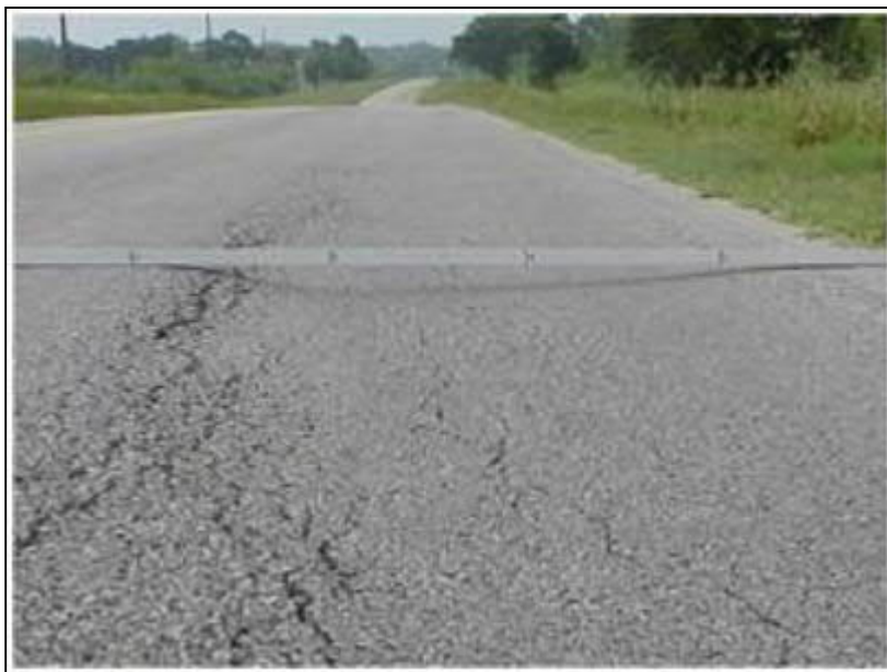
Figure 1.3.2-3: Roadway Rutting
