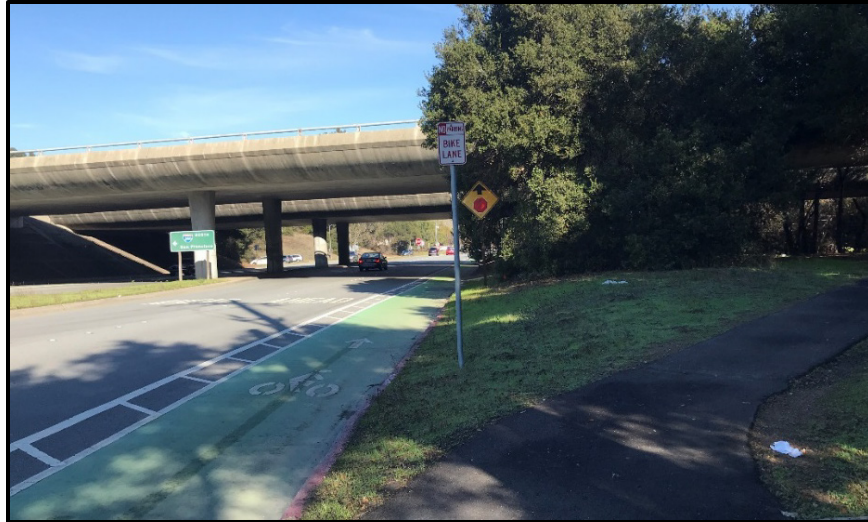
Photo 5: Alpine Road UC (L/R) Bridges; View eastbound of designated bike path and Alpine Trail
