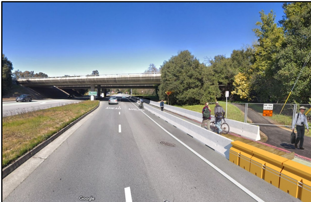
Photo 12: Simulation of the temporary detour path as described above for Alpine Trail during construction.
