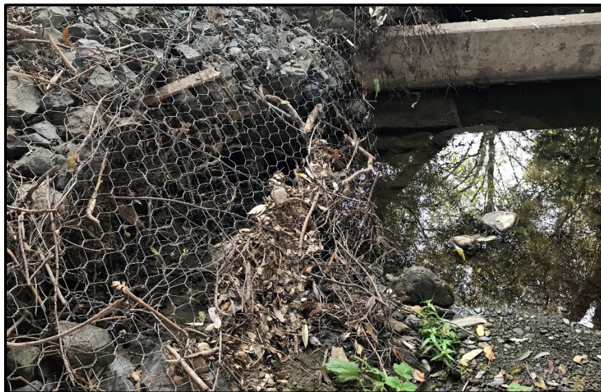
Photo 4: Alpine Road UC (L/R) Bridges; View south east of the gabion mattress (left side) and a weir (right side)
