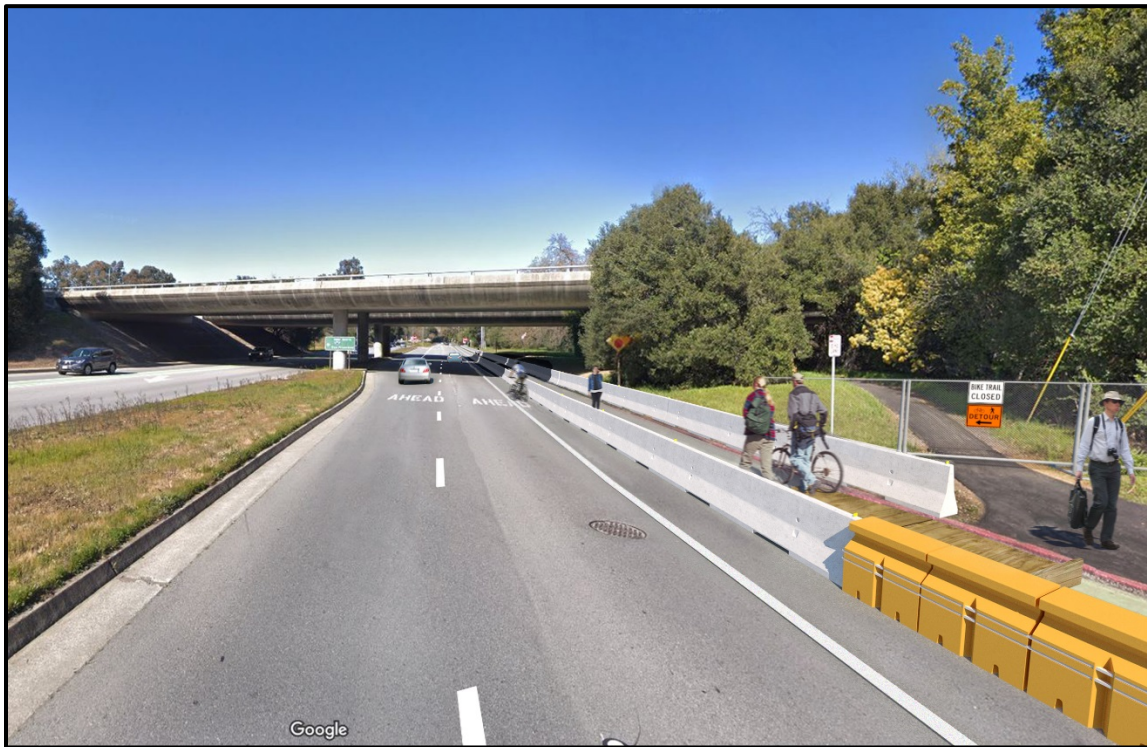
Photo 11: Visual Simulation of the temporary detour path as described above for Alpine Trail during construction.
