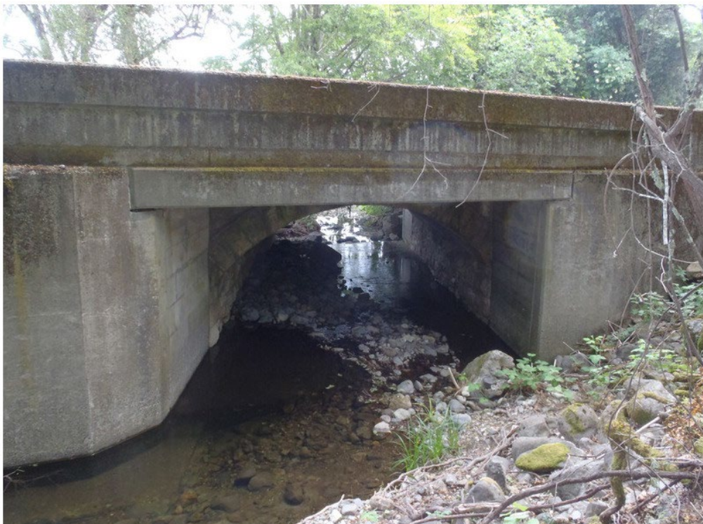
Figure 1-4 Upstream View of Bridge Opening
