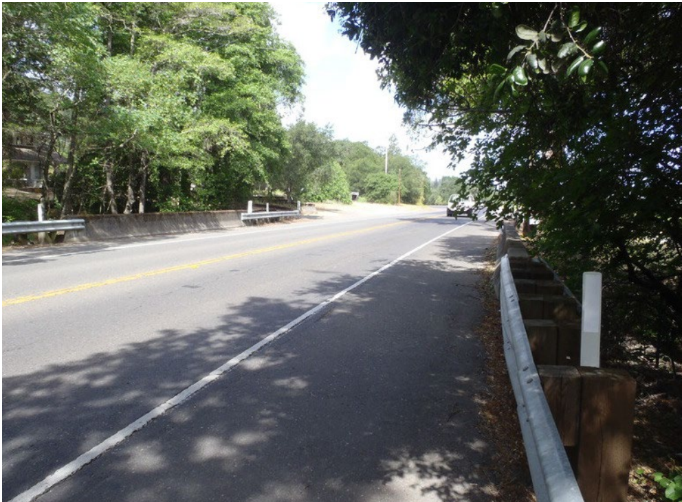
Figure 1-3 Northbound View of Existing Bridge
