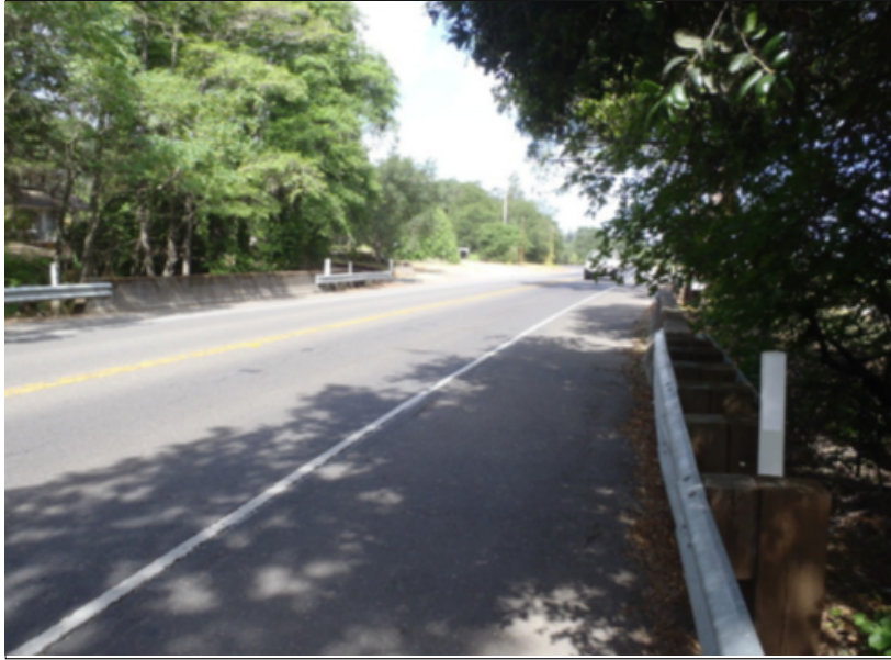
Existing view of Ritchie Creek bridge from northbound SR 29.
