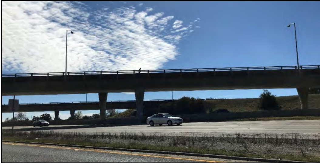
Photo 6: Sand Hill Road OC (South and North) Bridges; view looking southeast
