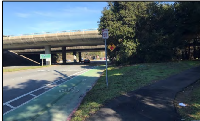
Photo 2: Alpine Road UC (L/R) Bridges; View eastbound of designated bike path and Alpine Trail
