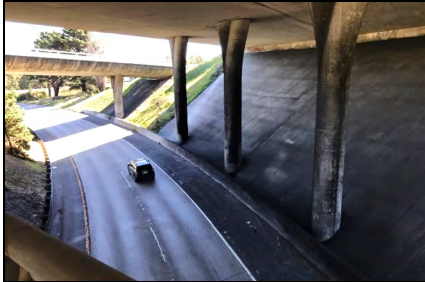
Photo 9: I-280/I-380 Separation Bridge; View of EB I-380 from a staging area under the I-280 Bridge
