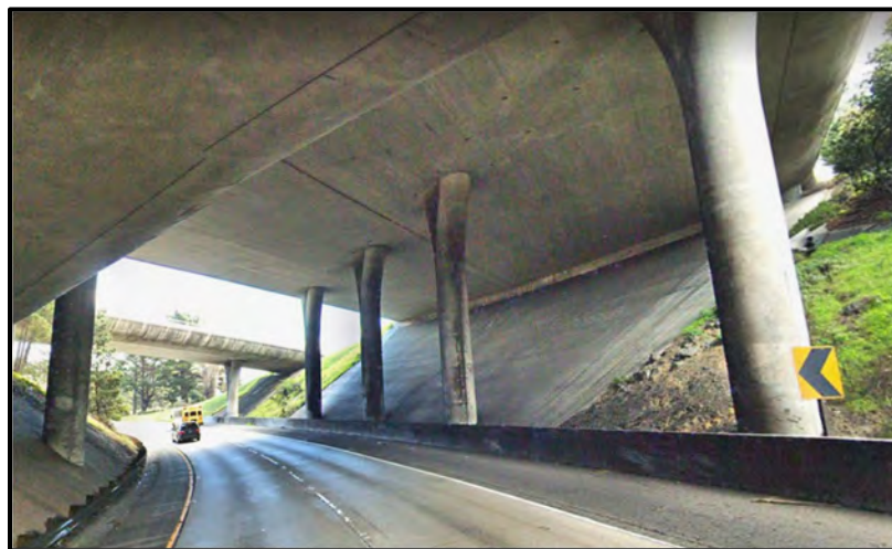
Photo 8: I-280/I-380 Separation Bridge; View from EB I-380 of Bent 3 and Bent 2 of the (I-280) Bridge. Slope paving is visible on the right side of the image behind the columns.
