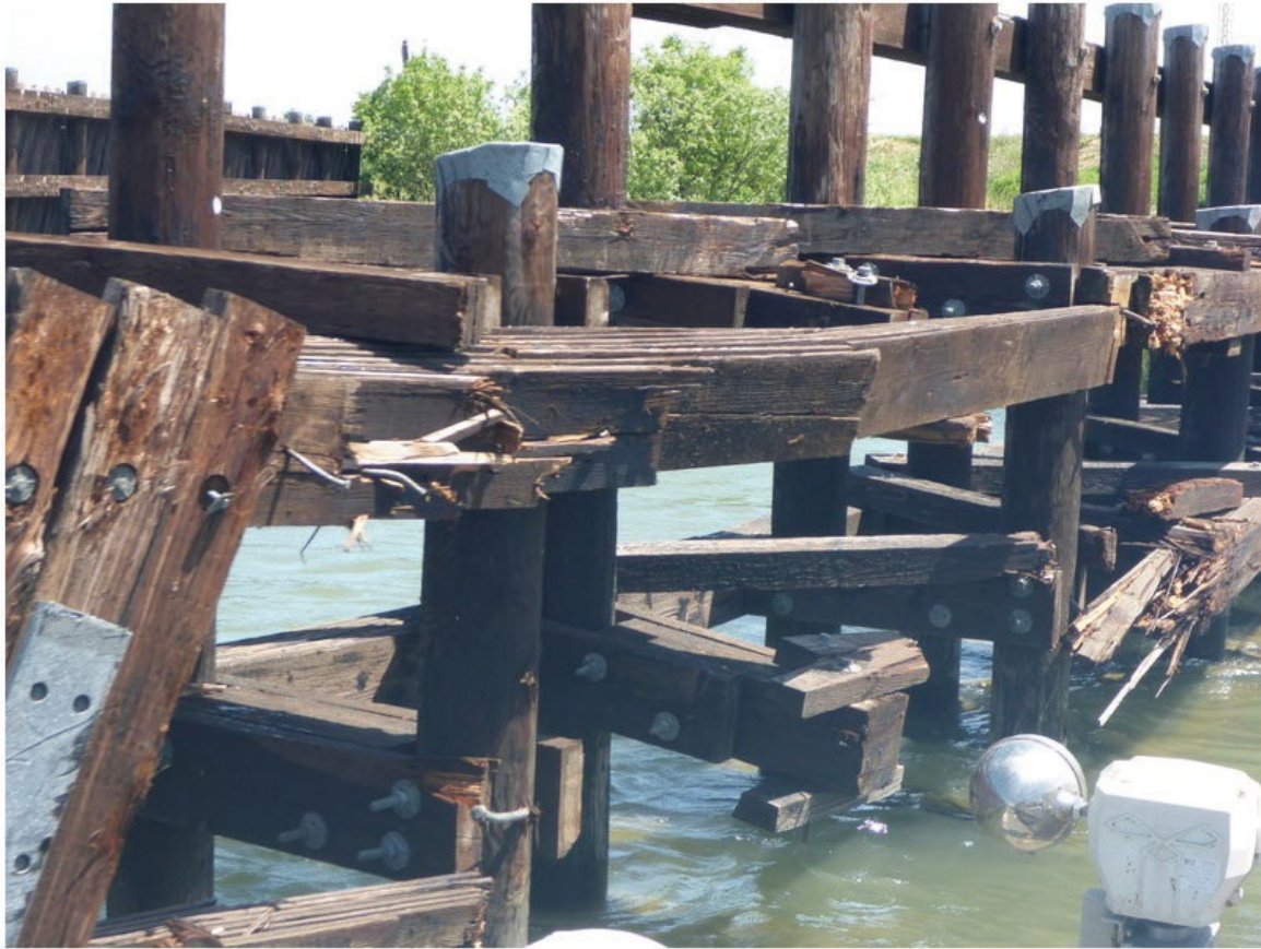
Figure 1-3. Existing Fender System on Ryer Island
