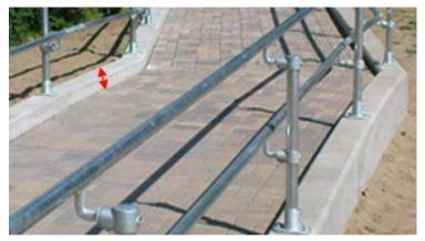
□ \*Exception – A curb or barrier is not required where a guard or handrail is provided with a guide rail centered 2 inches minimum and 4 inches maximum above the surface of the ramp.
