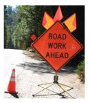
Each advance warning sign in each direction of travel must be equipped with at least two flags for daytime closures. Each flag must be at least 16by-16 inches and must be orange or fluorescent red-orange. Flashing beacons must be placed at the locations indicated for lane closures during hours of darkness.
