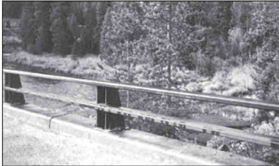
This Wyoming Rail from Virginia is a good example of the reason for a see-through rail. The rail is also suitably unassuming.
