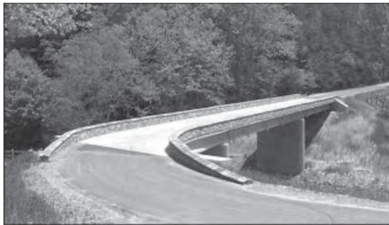
Most of the unique designs were located in scenic areas where traffic speeds and traffic counts are quite low. This stone railing from Kentucky is a good example.
