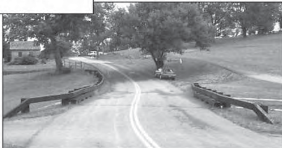
This culvert bridge is located near a golf course in Kentucky but is interesting for its craftsmanship and ingenuity. This is a steel-backed timber railing.
