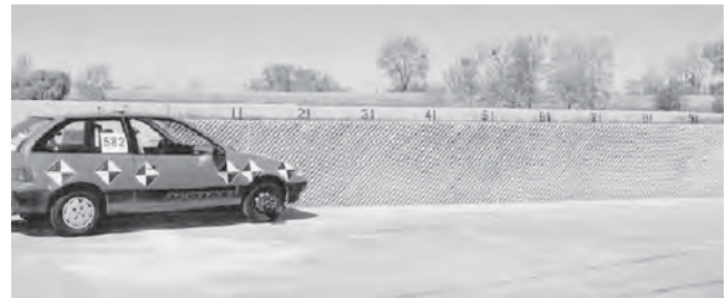
Figure 33. Caltrans single-slope barrier with fluted surface texture.
