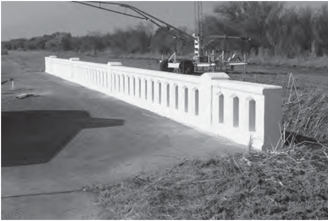
Figure 42. Texas T411 aesthetic bridge rail.
