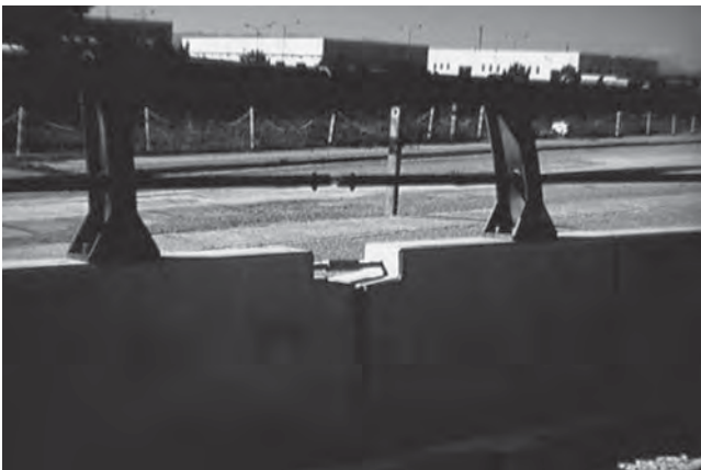
Figure 6. New Jersey border bridge used in Italy.
