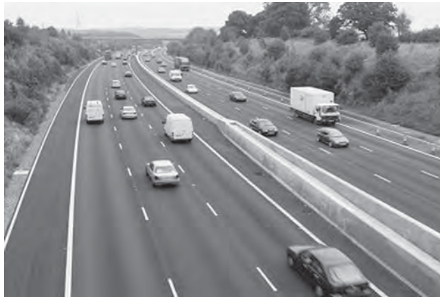
Figure 7. Concrete barriers used in the United Kingdom.
