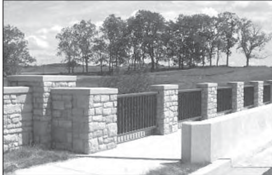
Special railing designs such as this one from Kentucky are typically associated with pedestrian access and always protected by a crashworthy wall.
