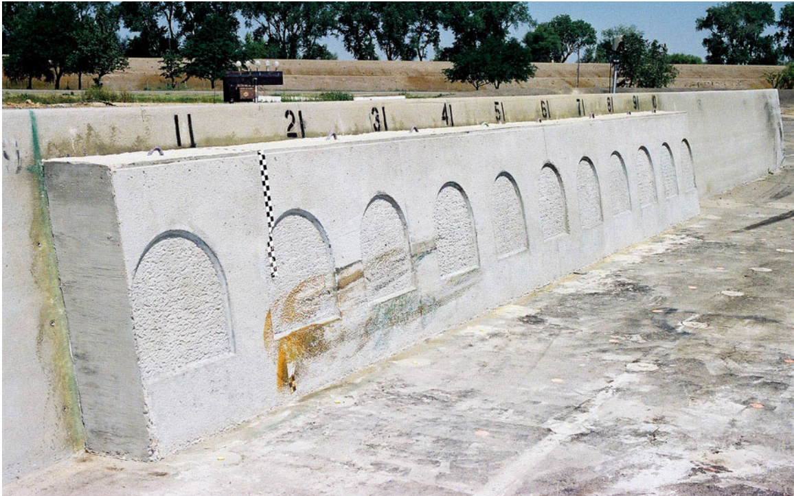
Figure 2-29 Test article after Test 584
