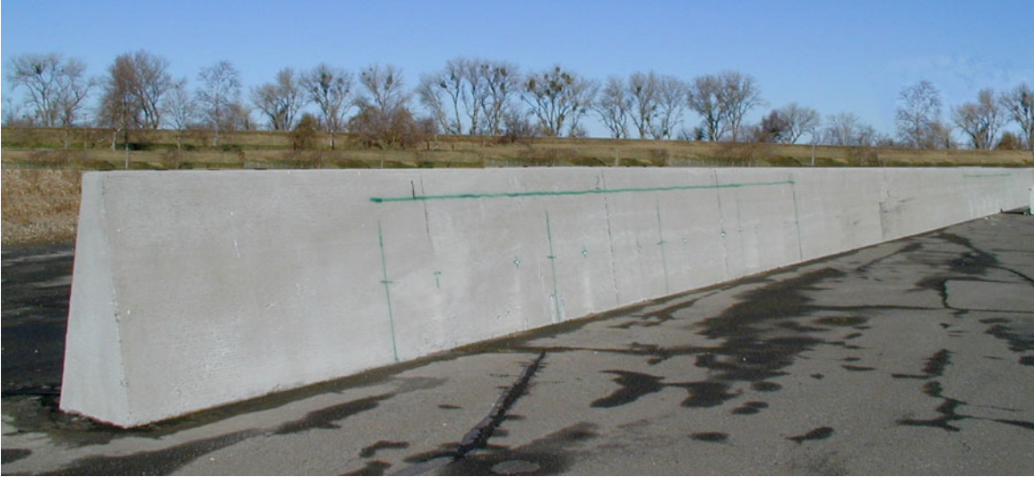
Figure 2-1 Existing Type 60G barrier
