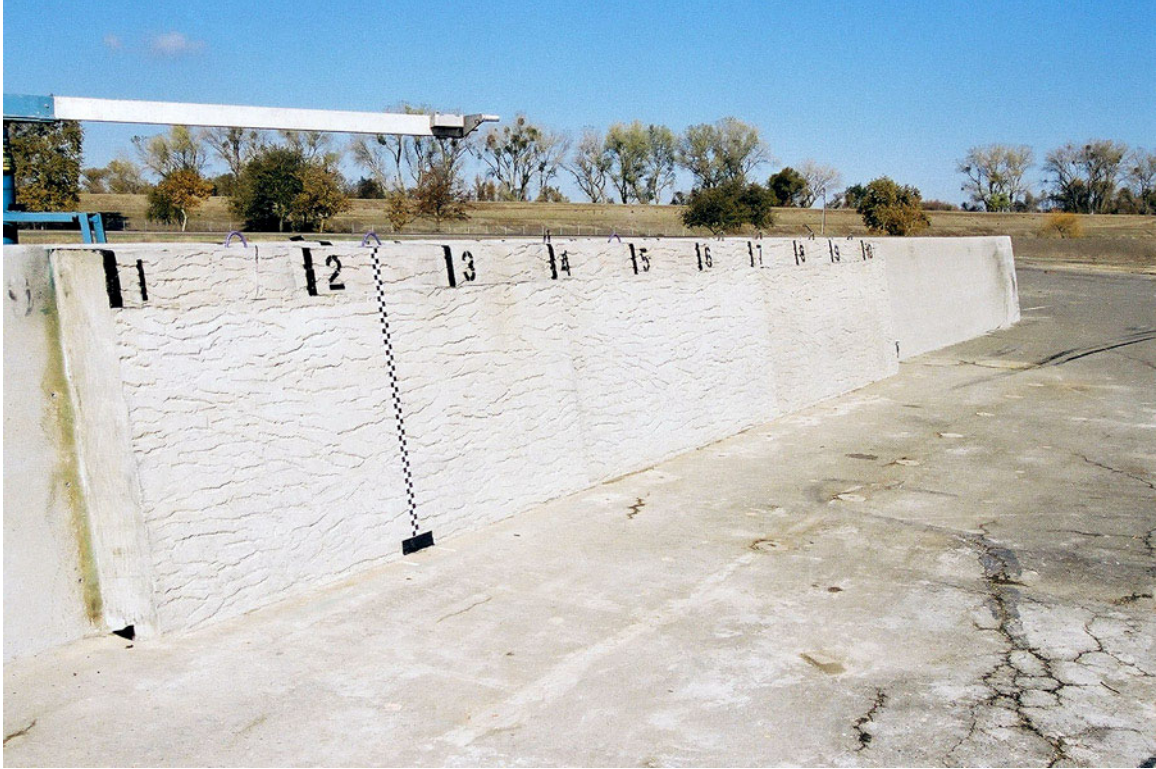
Figure 2-51 Fractured Granite test article prior to Test 588
