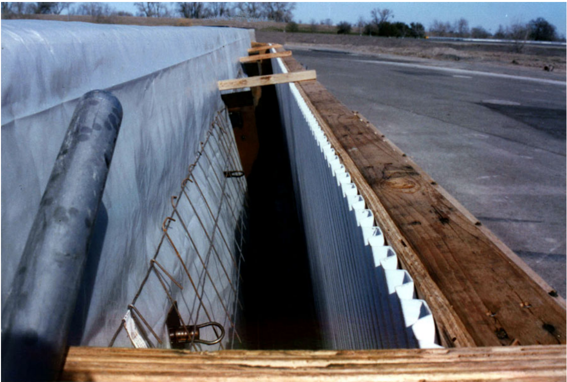
Figure 2-2. Formwork ready for concrete placement (note the plastic sheeting and ferrule loop inserts)
