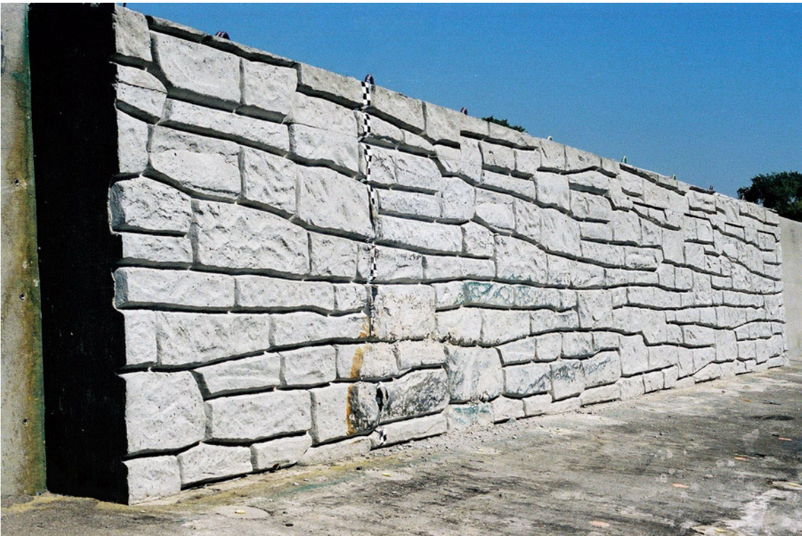
Figure 2-44 Drystack test article after Test 587
