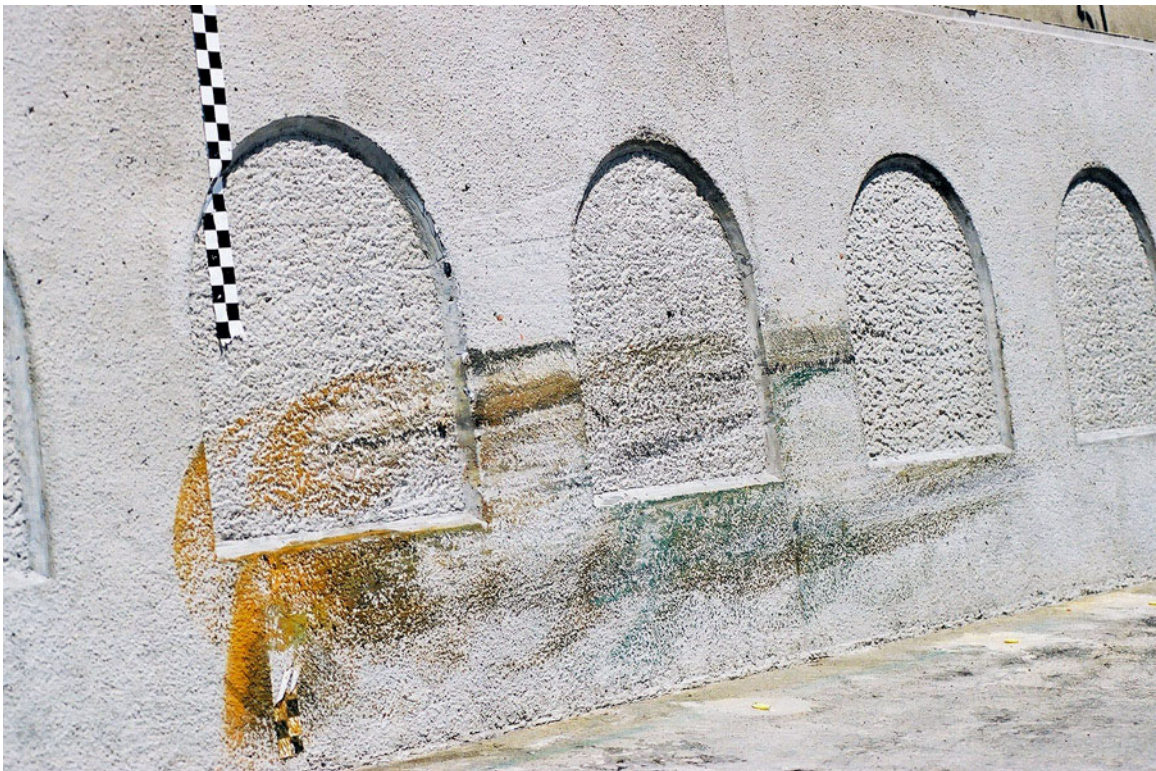
Figure 2-30 Test article after Test 584
