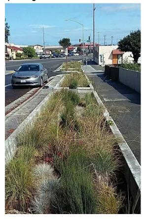
Figure 8-L – Bioretention features separate modes on SR-123 in El Cerrito
