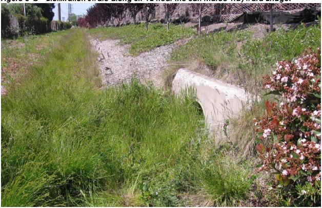
Figure 8-P - Biofiltration swale adjacent to I-5 in San Diego
