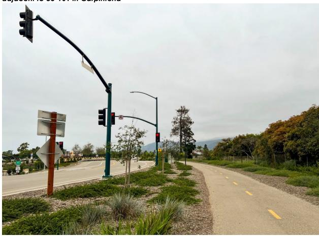
Figure 5-K – A raised Class IV separated bikeway connects to an overcrossing over US-101 in Belmont
