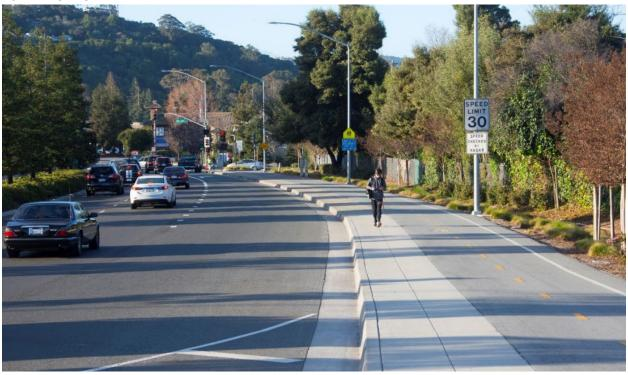
Figure 5-L - Delineators provide vertical separation on a suburban segment of SR-126 in Fillmore
