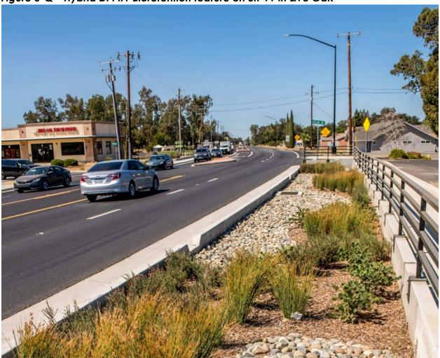
Figure 8-R – Arid climate DPPIA utilizing aggregates on SR-14 near Santa Clarita
