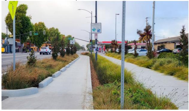
Figure 8-M – Climate-adapted plant material in a median bioretention feature at the Palomar Transit Center in Chula Vista
