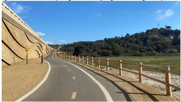
Figure 5-C - Class I bikeway along I-5 and San Elijo Lagoon in San Diego County
