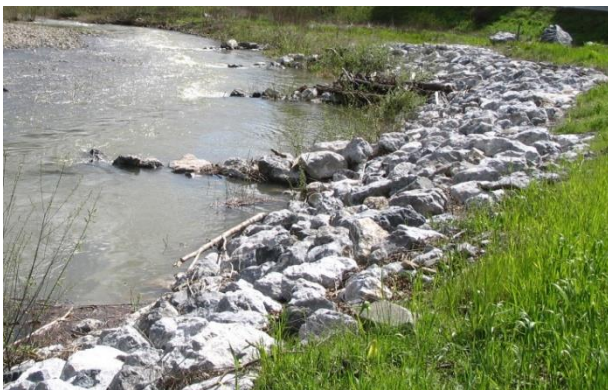
Bendway weirs in conjunction with rock slope protection.
