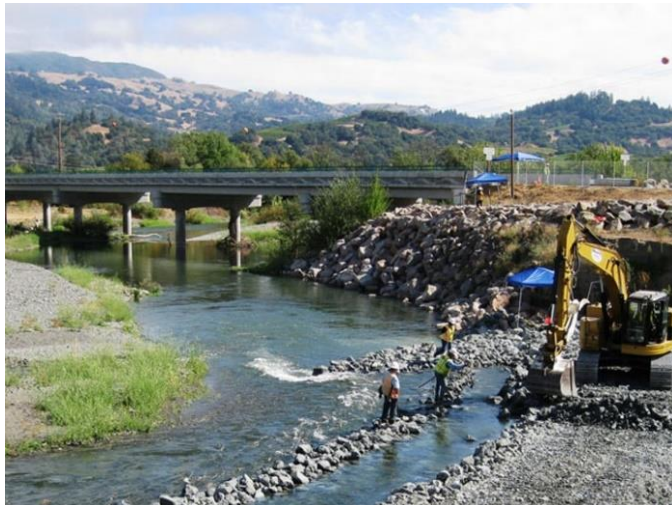
Longitudinal Peaked Stone Toe Protection (LPSTP) with Rock Vanes for Chinook Salmon Habitat Enhancement, Route 128, Russian River Bridge in Geyserville
