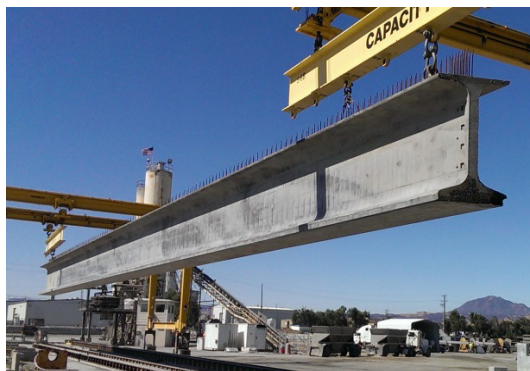
B) Pretensioned wide-flange girder
