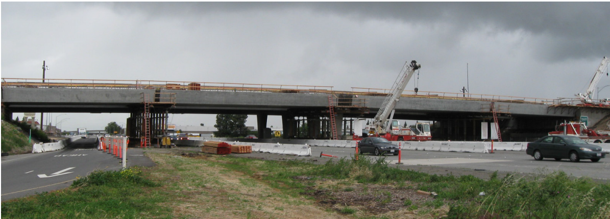
Figure 5.3.3-8 Precast Bath-tub Girder Segments Spliced Near Midspan Using Temporary Supports at Harbor Blvd. Overcrossing (Bridge No. 22-0108, Caltrans)
