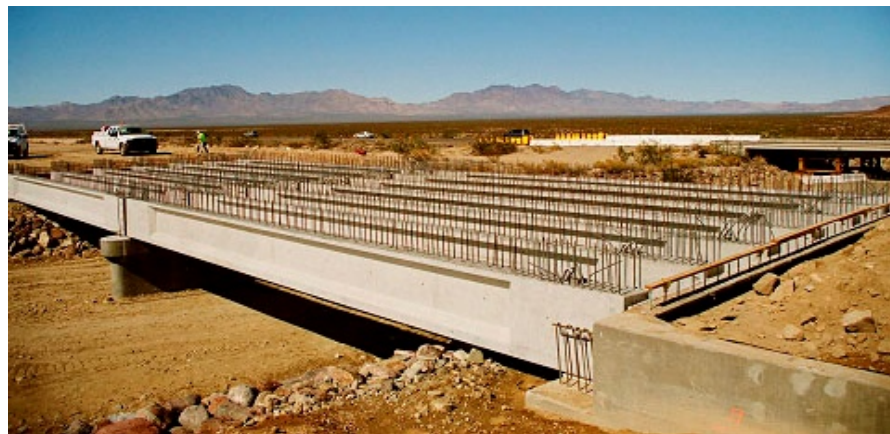
Figure 5.3.3-2 Drop Cap at Chuckwalla Wash Bridge (Bridge No. 54-1278L, Caltrans)
