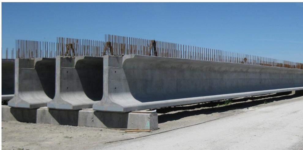
Figure 5.3.2-2 California Wide-Flange Girders
