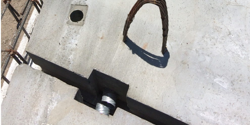
Figure 5.4-6 Transverse Diaphragm Breakout, Courtesy of Confab, CA
