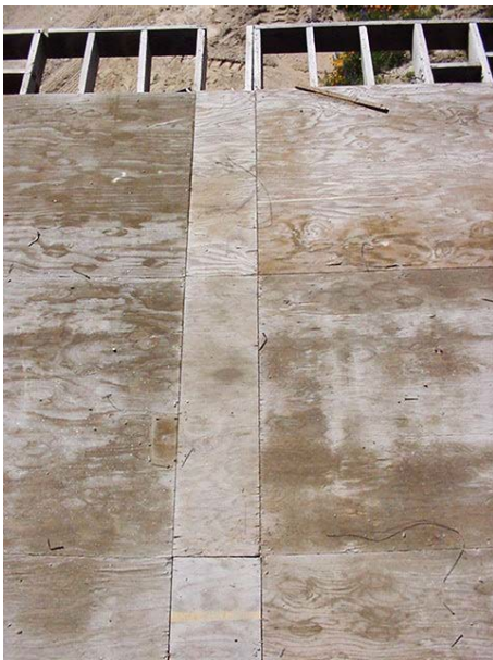
Figure 2. Form Filler Strip of Plywood
