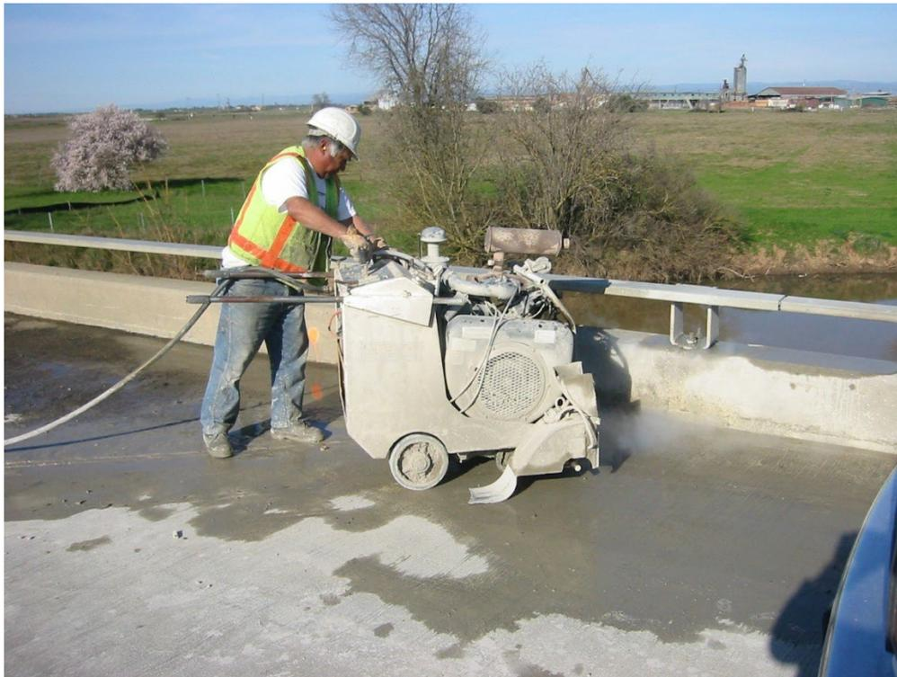
Figure 3-6. Water Cooled Concrete Saw
