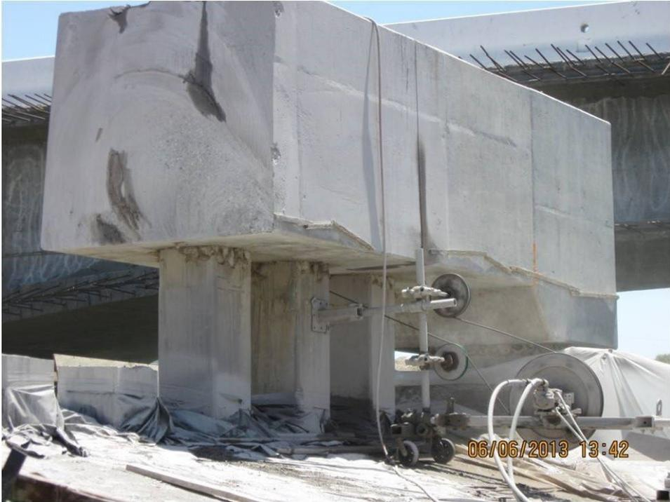
Figure 3-8. Diamond Wire Saw, Colorado River
