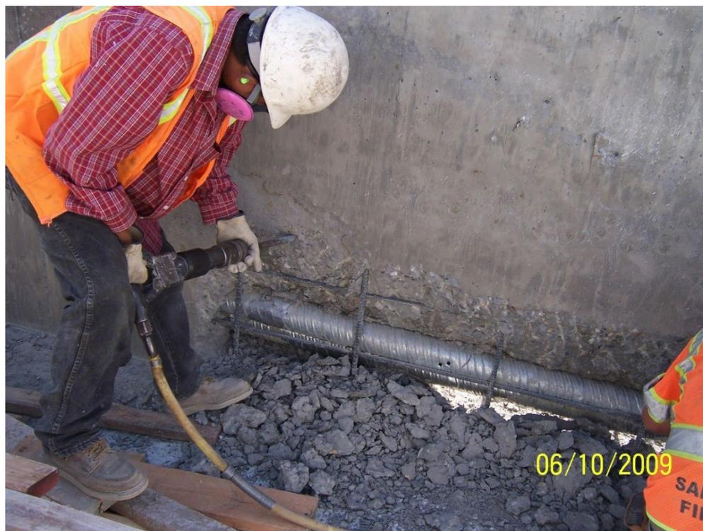
Figure 3-9. Handheld Pneumatic Hammer, Bear River
