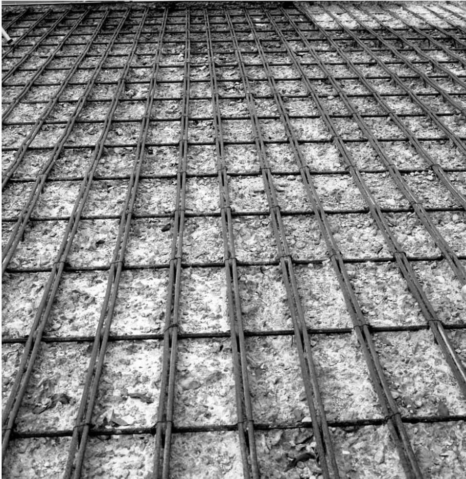
Figure 3-12. Hydroblasting for Partial Deck Removal
