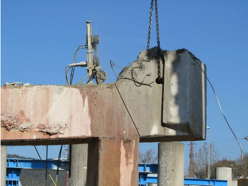
Figure 3-7. Diamond Wire Saw
