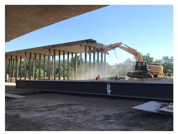
Figure 6-23. Weakening Pile Extensions for Span by Span Removal, Simmerly Slough
