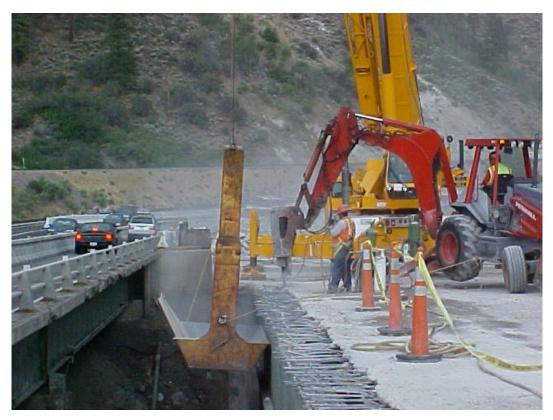
Figure 6-3. Custom Debris Box used for Edge of Deck Removal
