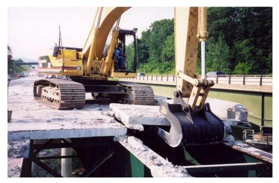
Figure 6-9. Slab Removal Attachment on Excavator
