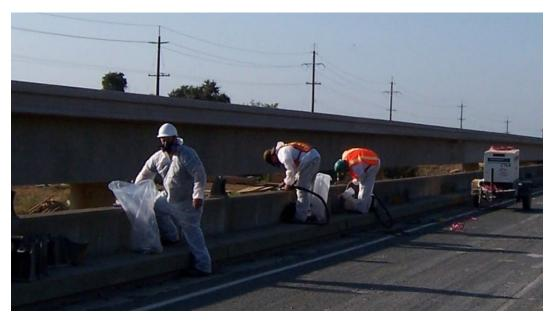
Figure 6-4. Asbestos Shim Removal
