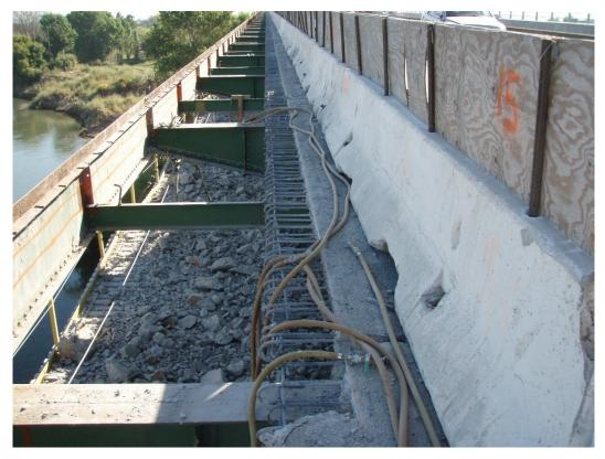
Figure 6-6. Suspended Debris Containment Platform
