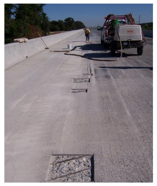
Figure 6-14. Unsound Concrete Removed for Repair After Asphalt Surfacing Removal
