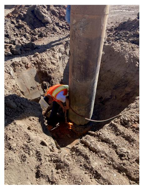
Figure 6-27. Piling Removal Below Grade, Simmerly Slough
