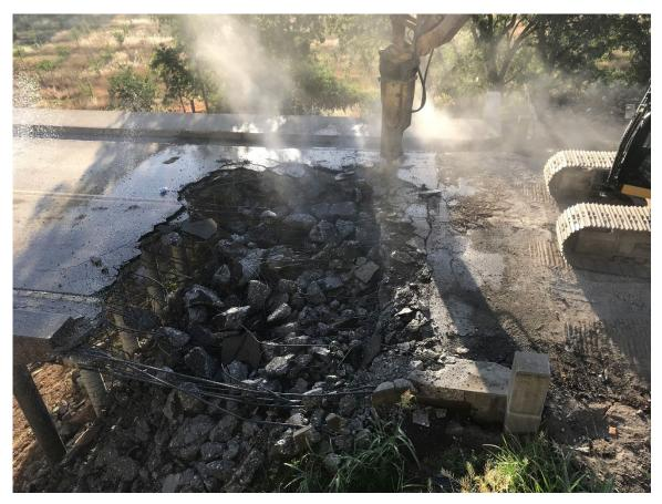
Figure 6-11. Slab Deck Removal, Simmerly Slough
