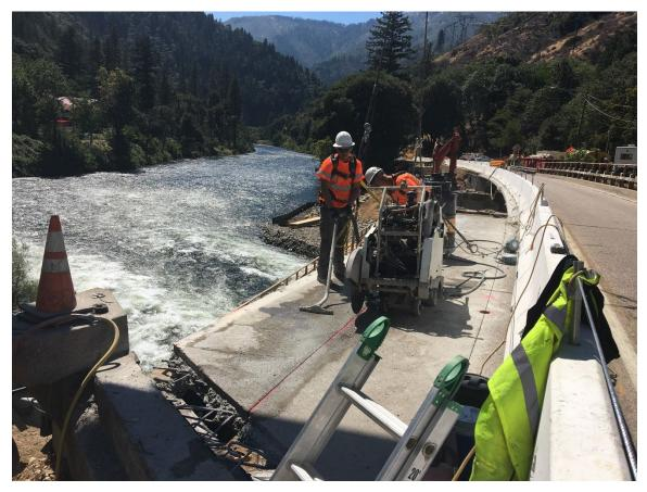
Figure 6-8. Sawing Deck for Removal, Yellow Creek
