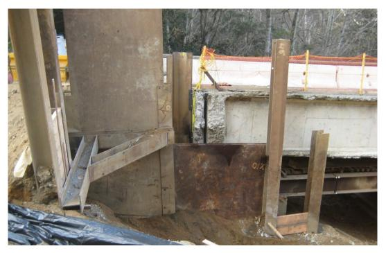
Figure 6-25. Partial Abutment Removal with Shoring and Temporary Support, Greenwood Creek
