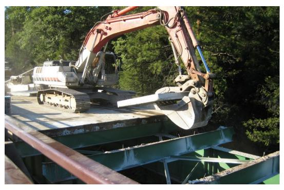
Figure 6-10. Slab Removal with Bucket and Thumb on Excavator, Spanish Creek
