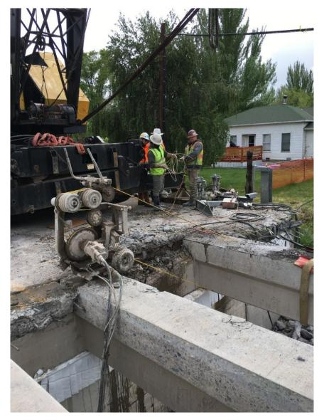
Figure 6-19. Wire Saw Cutting Concrete Girder Supported by a Crane
