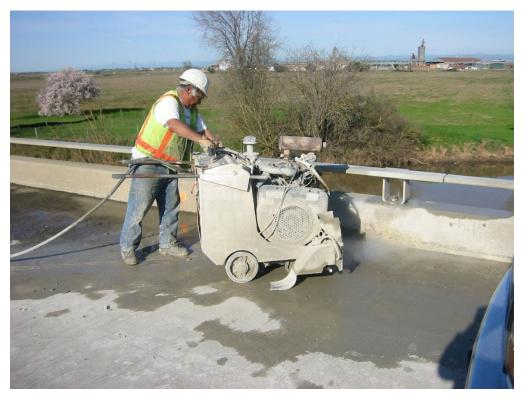
Figure 3-6. Water Cooled Concrete Saw
