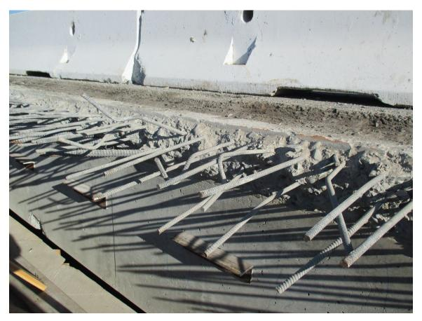
Figure 6-13. Sawcut Line and Reinforcement Preservation for Widening, Sacramento
