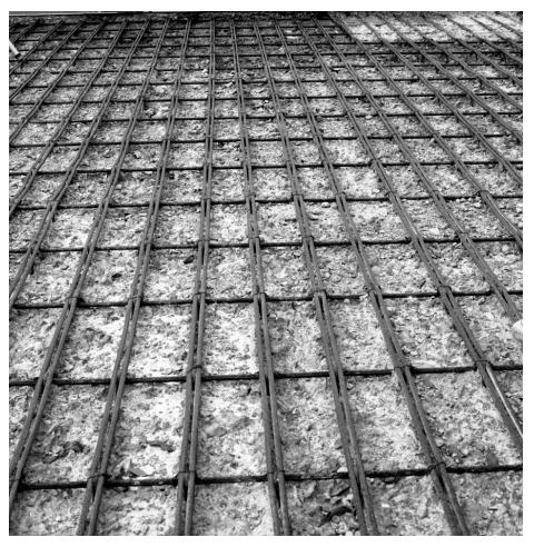
Figure 3-12. Hydroblasting for Partial Deck Removal
