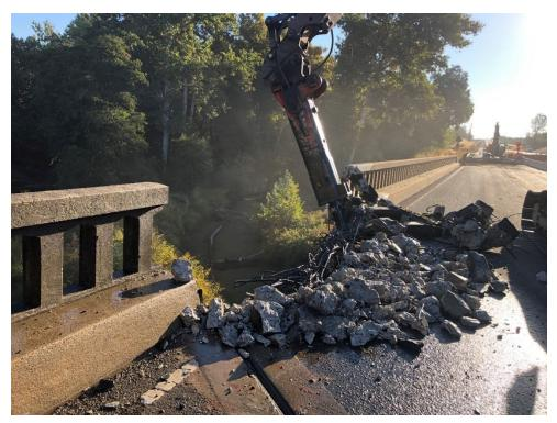
Figure 6-7. Barrier Rail Removal, Dry Creek
