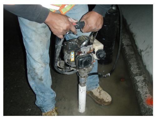
Figure 6-15. Coring Drainage Hole Through Deck
