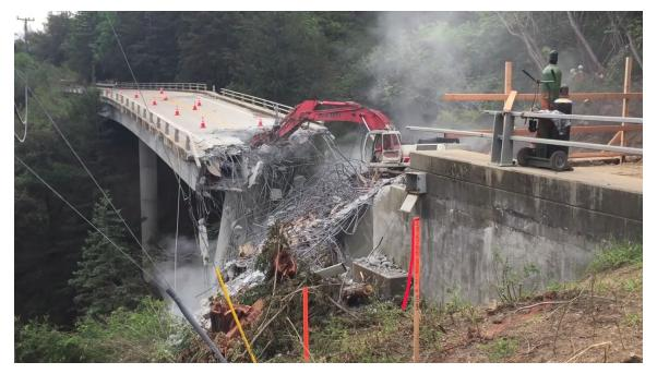
Figure 6-28. Special Bridge Removal at a Partially Collapsed Bridge, Pfeiffer Canyon
