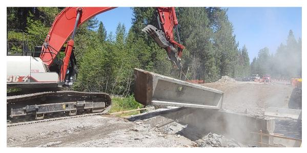
Figure 4-4. Precast Girder Removal with Excavator, Hat Creek
