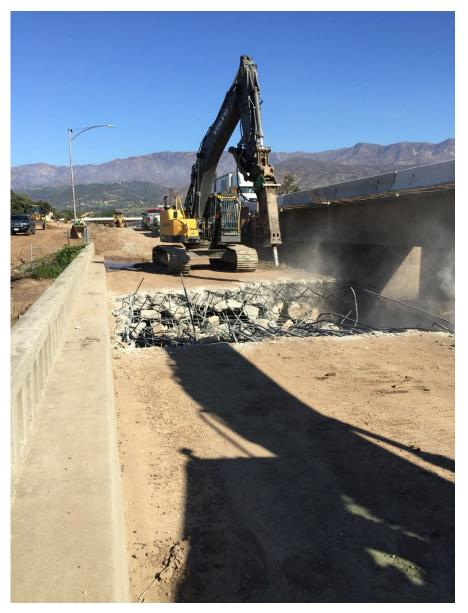
Figure 4-2. Typical Equipment Live Load, Carpinteria Creek
