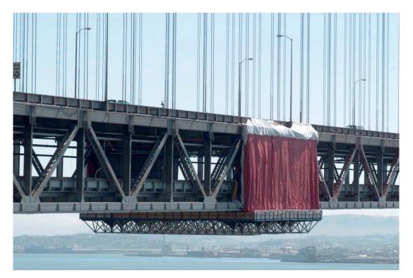
Figure 3-20. San Francisco-Oakland Bay Bridge Retrofit Included Partial Bridge Removal on a Suspension Bridge
