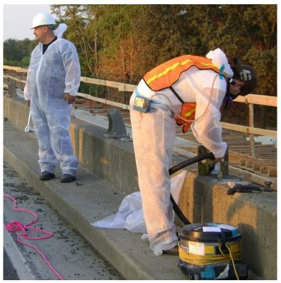
Figure 7-6. Asbestos Shim Removal from a Bridge Rail
