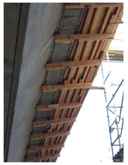
Figure 5-5. Four-Foot-Wide Protective Cover for Rail Removal, Sacramento
