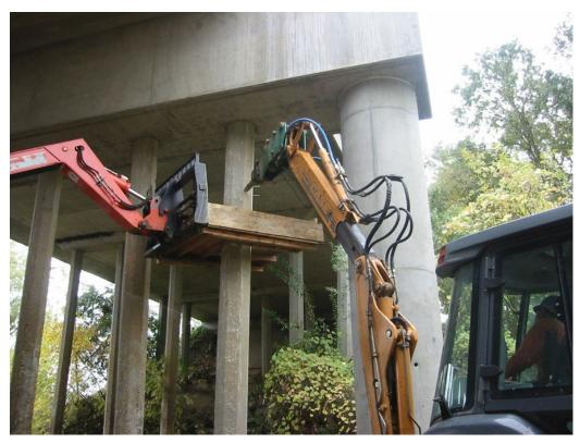
Figure 7-2. Debris Containment Platform, Honcut Creek
