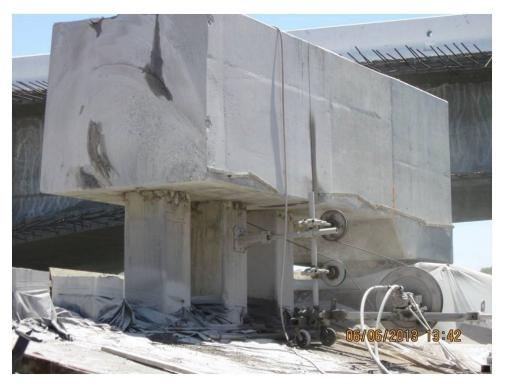
Figure 3-8. Diamond Wire Saw, Colorado River
