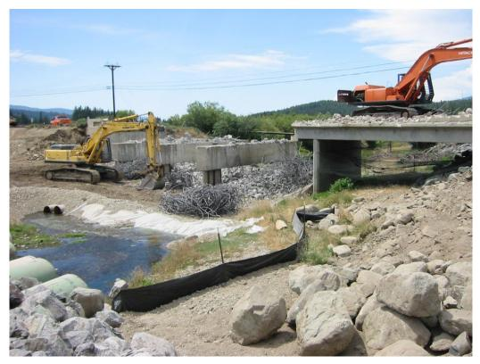
Figure 7-1. Clear Water Diversion Through Culverts with Bridge Removal on Gravel Pad, Sulpher Creek
