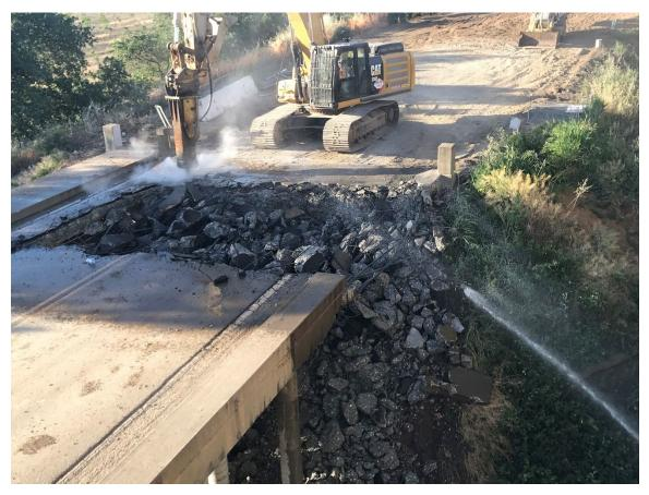
Figure 7-7. Water Applied to Control Dust, Simmerly Slough
