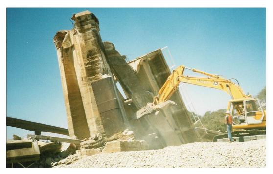
Figure 6-21. Pier Rotation After One Span of 4-Span Arch was Demolished
