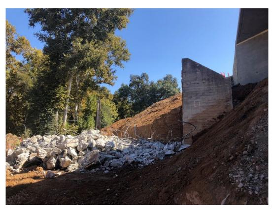
Figure 6-24. Abutment Removal, Dry Creek
