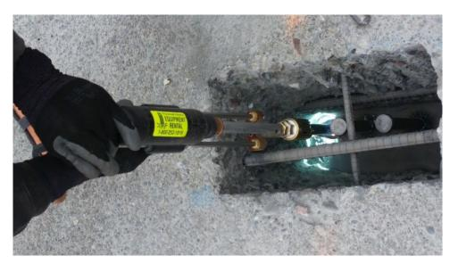
Figure 6-16. Installing Shear Studs on Steel Girders after Partial Removal of Concrete Bridge Deck
