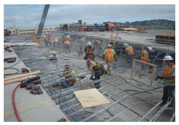
Figure 8-2. Workers Removing a Portion of a Hinge, San Francisco
