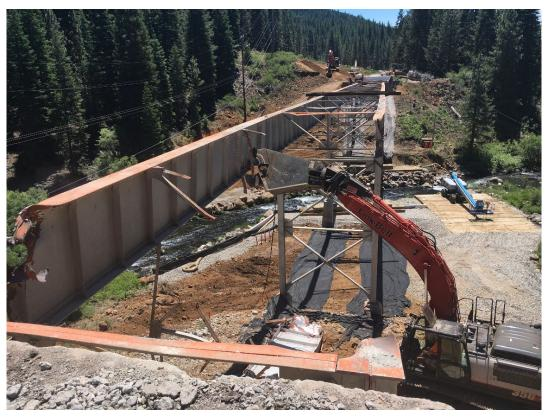
Figure 6-17. Excavator Mounted Hydraulic Shear Removing Steel Girder, Hamilton Branch
