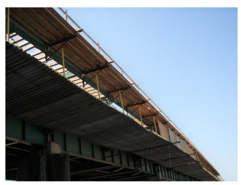
Figure 5-4. Suspended Scaffolding on Overhang for Debris Containment, Marysville
