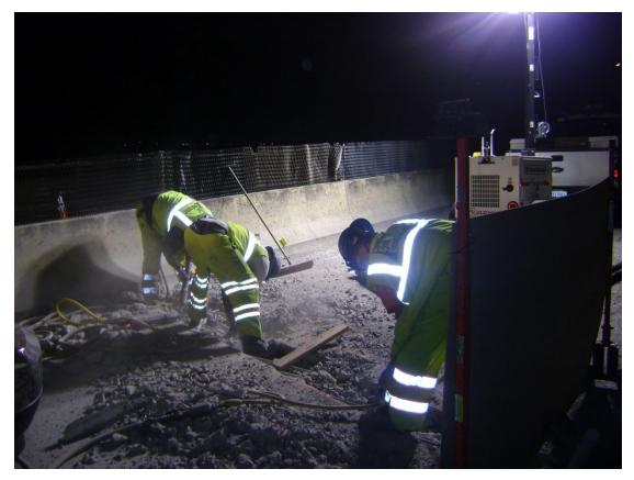
Figure 8-3. Repair of Bridge Joint at Night, Yuba River
