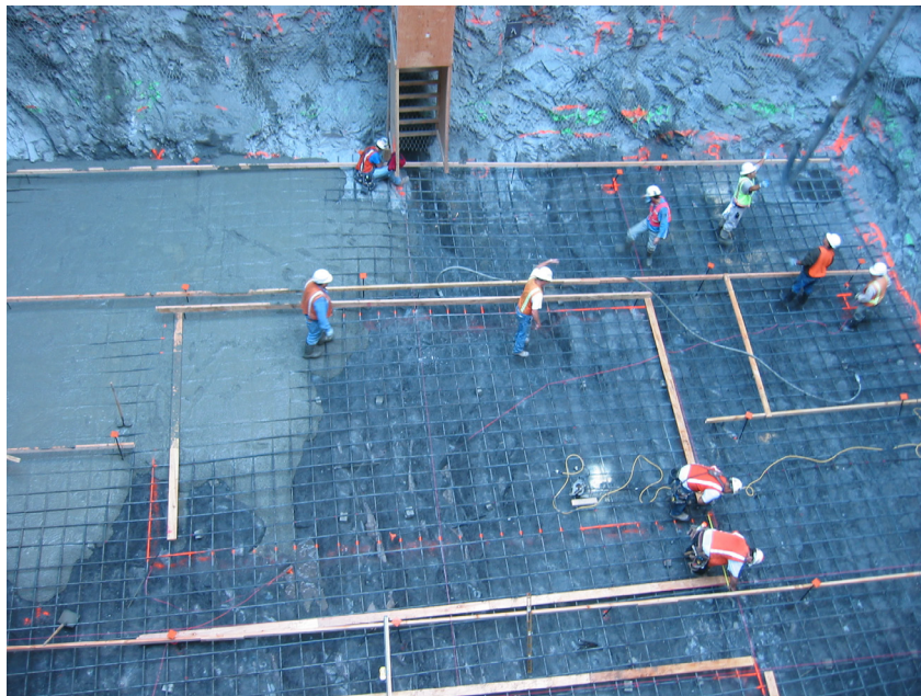
Figure 7-22. Start of Reinforcement / Cooling Pipe Layout W2 Anchor.
