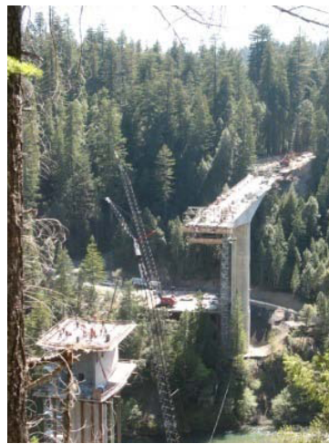
Figure 7-33. Confusion Hill Segmental Bridge.
