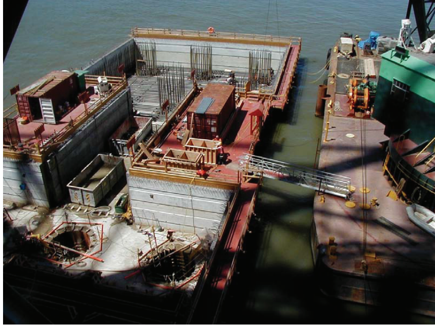
Figure 7-18. Footing or Pile Cap Prior to Placement of Mass Concrete.
