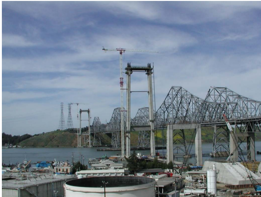
Figure 7-19. Zampa Bridge Anchor Blocks and Towers During Construction.
