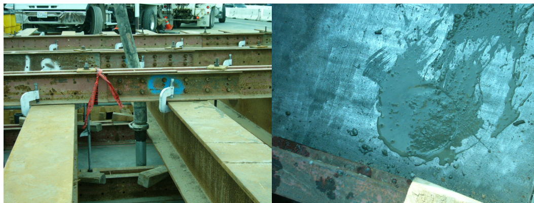
Figure 7-7. Concrete Pump Hose Connected to 2” Pipe and Grouted Pipe Delivery Void.
