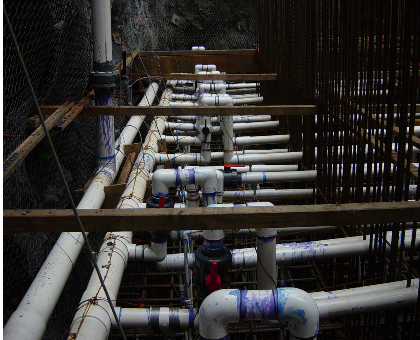
Figure 7-23. Complete PVC Cooling Pipe and Reinforcement Layout W2 Anchor.
