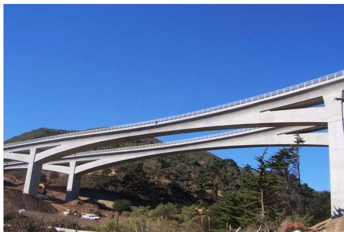
Figure 7-34. Devil's Slide Segmental Bridge.
