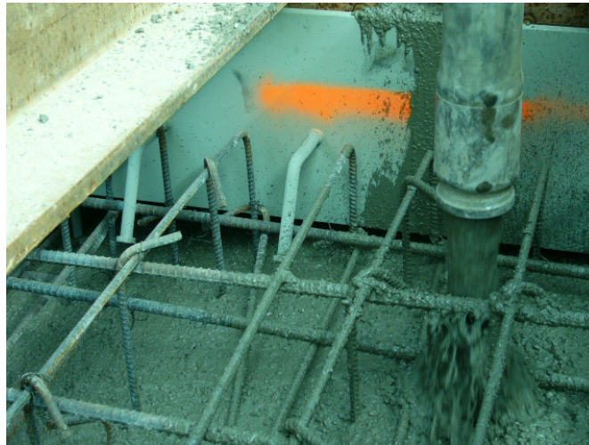
Figure 7-5. SCC Placement Tremie.
