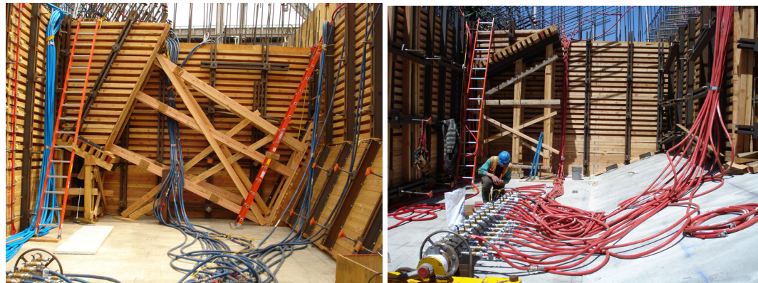
Figure 7-8. Forms for SCC Placement with Water-cooling Tubes.
