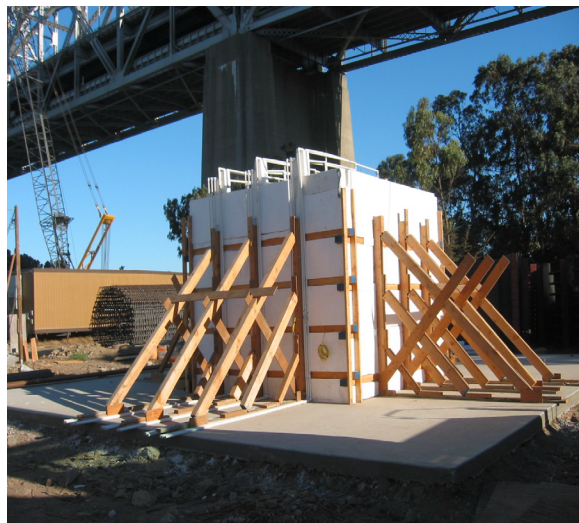
Figure 7-24. Footing Mock-up 10-ft Cube.
