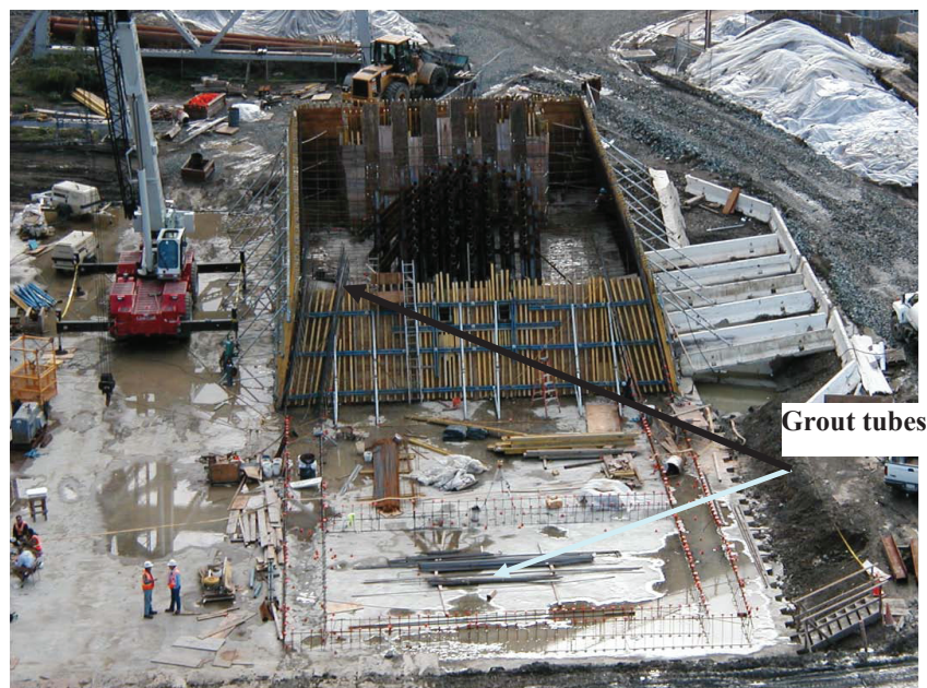
Figure 7-17. Anchor Block, Zampa Bridge.
