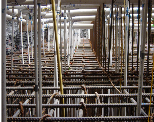
Figure 7-15. Cooling Pipes Tied to Reinforcing Steel.
