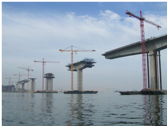
Figure 7-37. New Benicia-Martinez Bridge During Construction.
