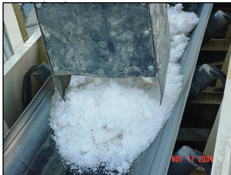
Figure 7-14. Batching Concrete with Ice.
