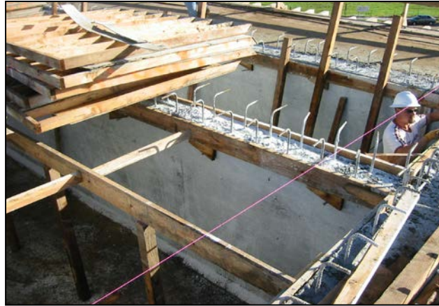
Figure 2.1-11. A String-Line Strung Between Deck Dowels.
