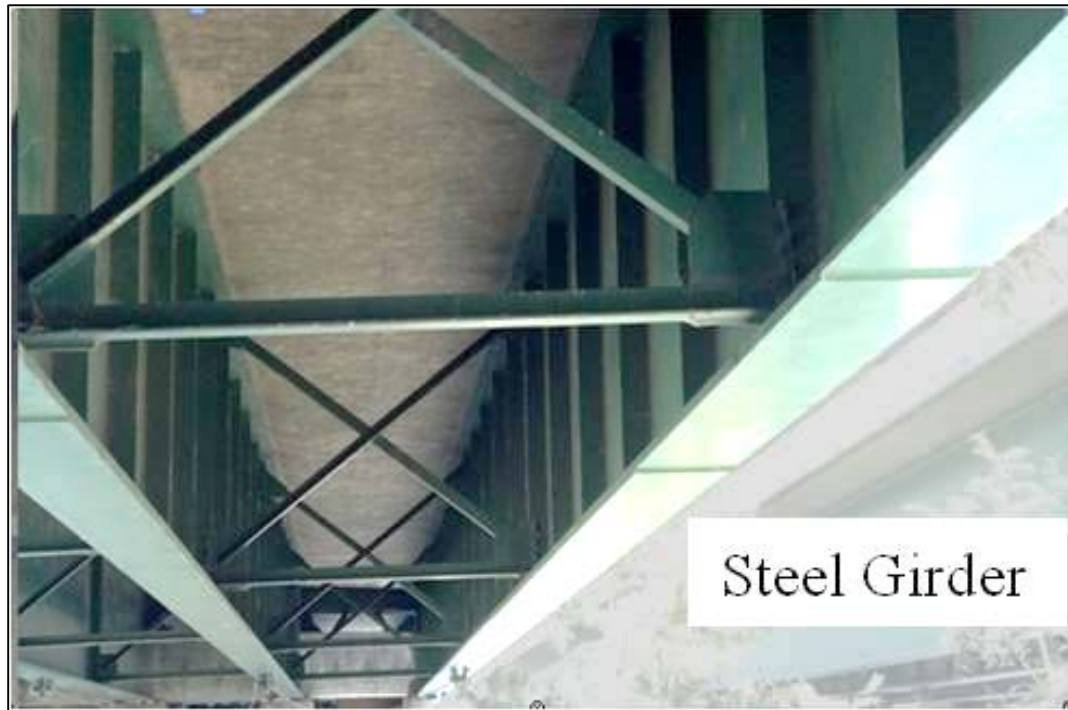
Figure 2.1-5. Example of a Steel-Girder Bridge.
