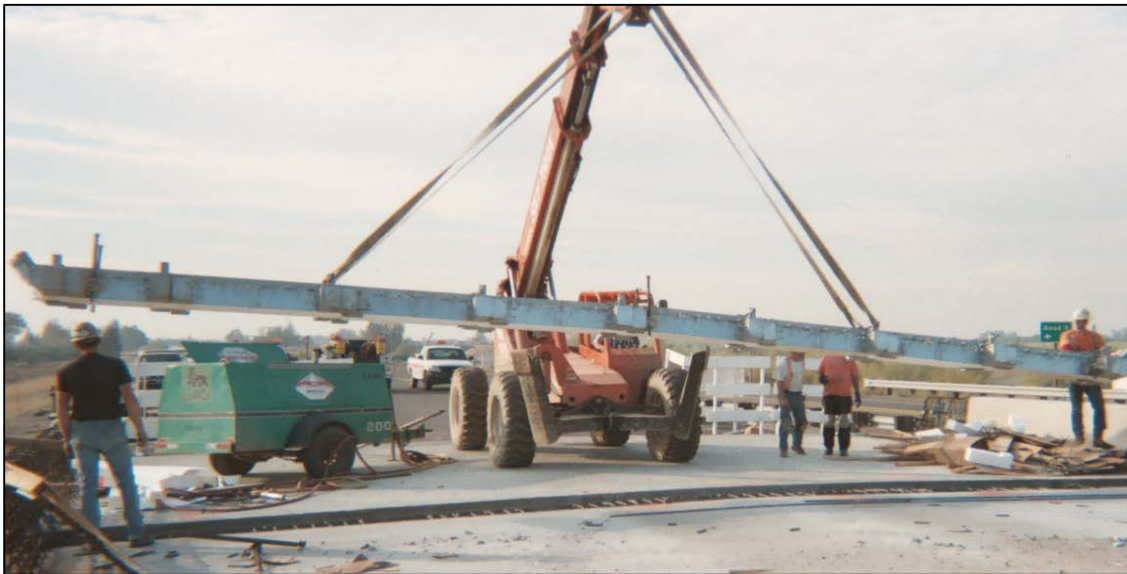
Figure 2.2-4. Joint Seal Assembly Installation.
