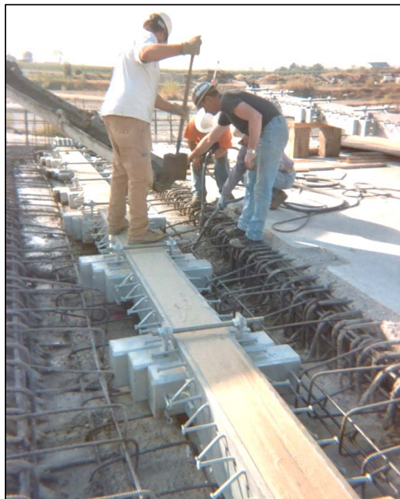
Figure 2.2-3. Threaded Spacer Rods Used to Hold the Correct Width.
