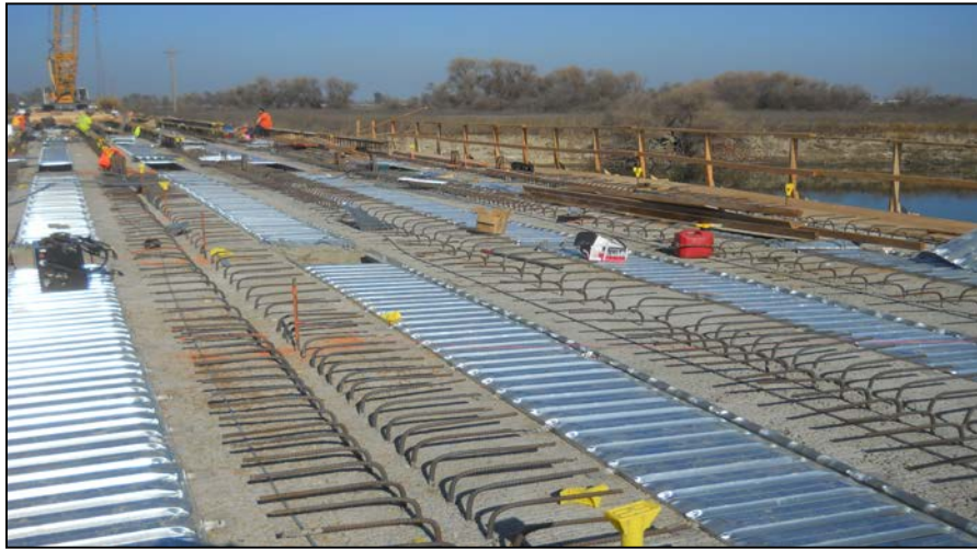
Figure 2.1-3. Stay-in-Place Metal Forming on a Precast Girder Bridge.
