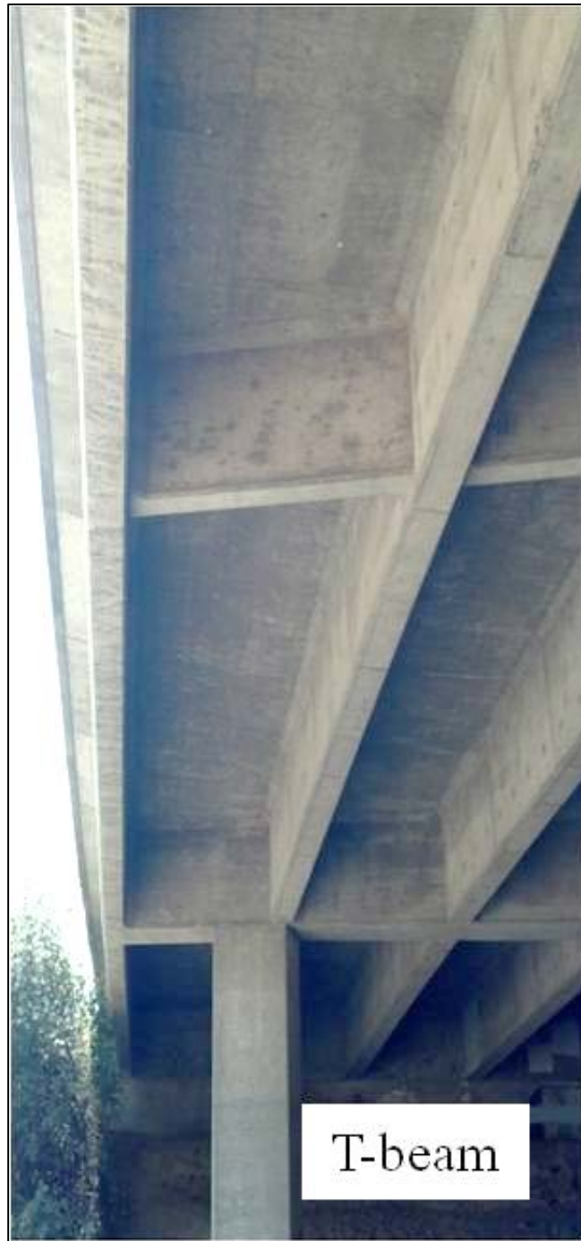
Figure 2.1-6. Example of a T-Beam Bridge.
