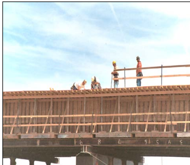
Figure 2.1-10. Overhang Post Supports Bearing Directly on the Falsework.
