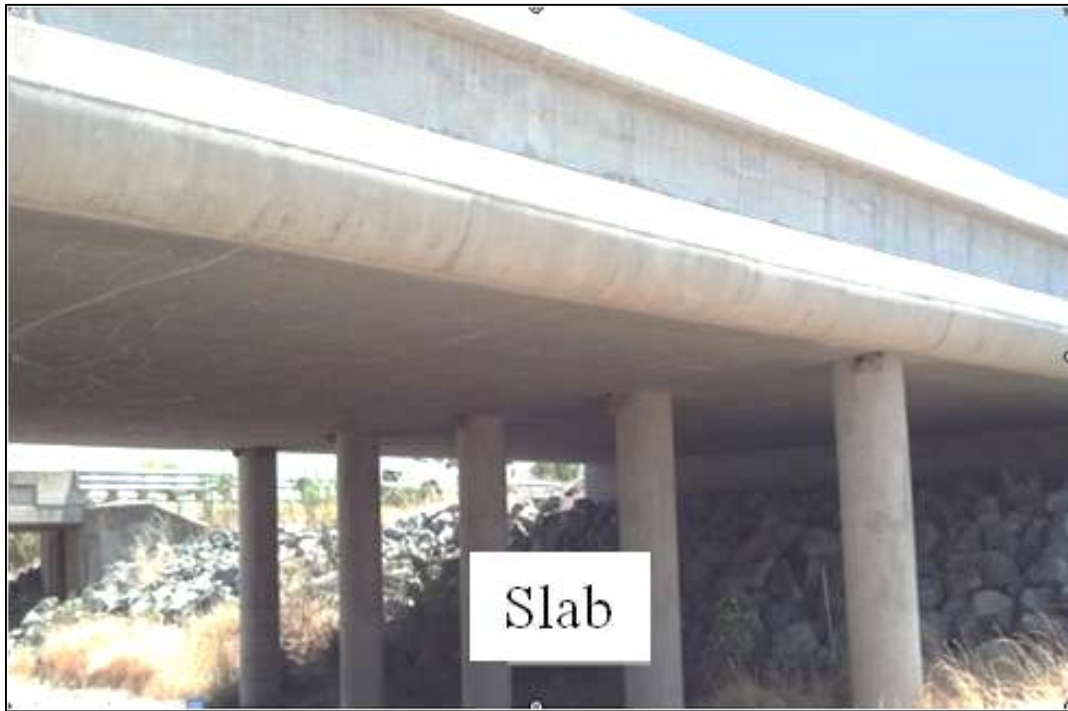
Figure 2.1-4. Example of a Slab Bridge.
