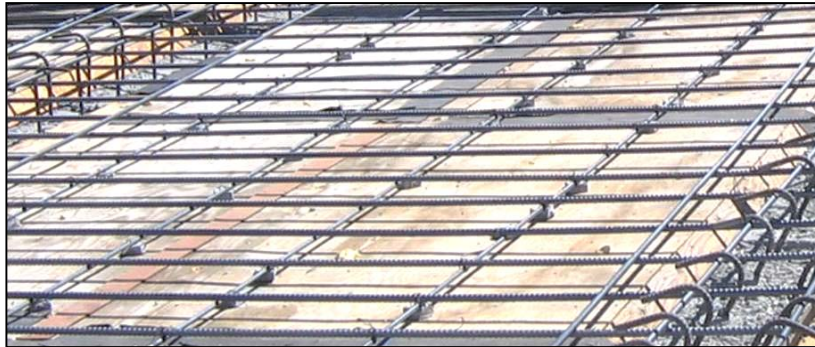
Figure 3.2-1. Precast Mortar Blocks Under the Bottom Rebar Mat.
