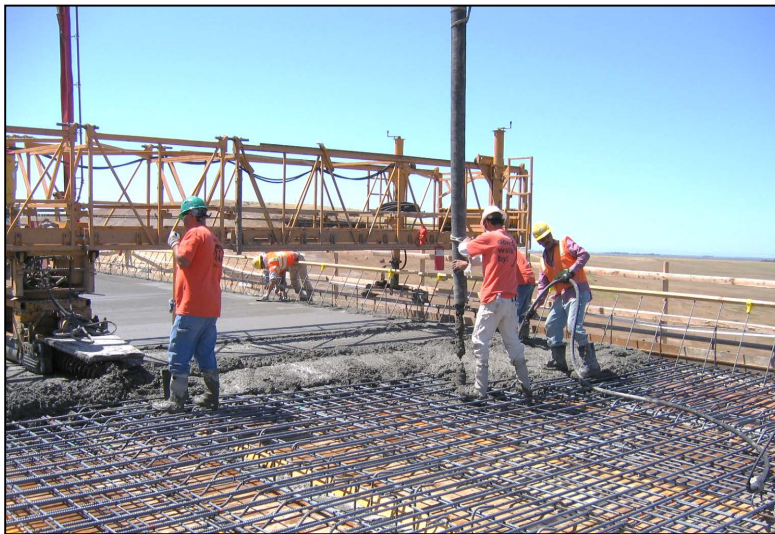
Figure 5.3-1. Vibrating Concrete.
