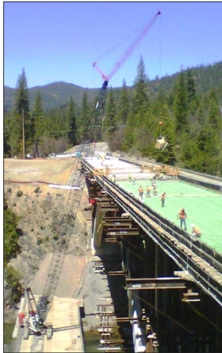
Figure 5.2-1. Crane and Bucket Concrete Placement.
