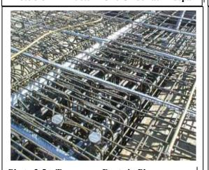
Photo 3-5 – Transverse Ducts in Place.
