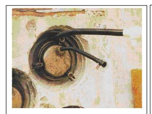
Photo 9-3 – Grout Cap and Tubes in Place.
