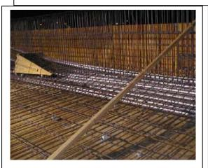
Photo 3-3 – 12 Ducts in One Girder at Midspan
