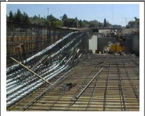
**Photo 3-4 – Part and Full Length Duct Profiles**
