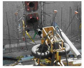
Photo 4-7 – Installation of Individual Strands by Pushing.
