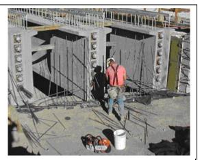
Photo A-2 – AVAR Spliced Girder Stressing.
