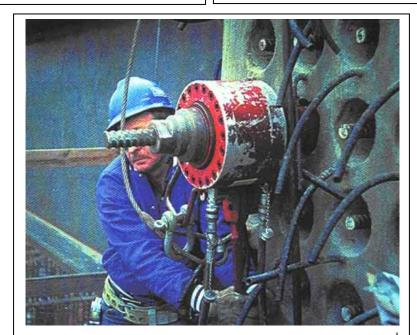
Photo 7-3 – High Strength Bar Stressing Operation.
