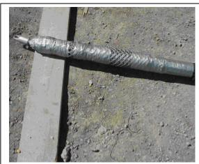
Photo 4-10 – Tendon Installed with Pulling Cuff
