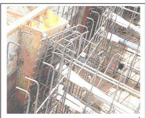
Photo A-4 – DSI Anchorages and Block-out.
