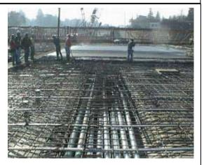
Photo 3-6 - Transverse and Longitudinal Ducts
