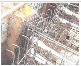
Photo A-4 – DSI Anchorages and Block-out.
