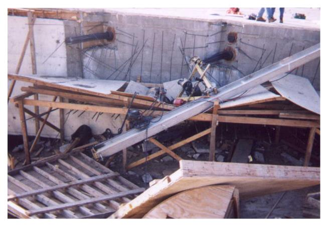
**Photo 1-1 – Example of Failure During Prestress Operations.**
