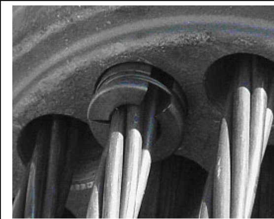
Photo 4-13 – Strand, Wedge, and Anchor Head
