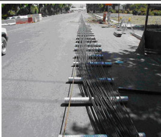
Photo 4-9 – Dirt Free Prestressing Tendon.
