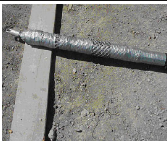
Photo 4-10 – Tendon Installed with Pulling Cuff
