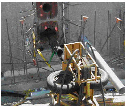
Photo 4-7 – Installation of Individual Strands by Pushing.
