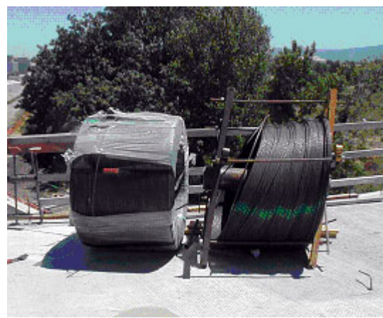
Photo 4-8 – Strand Packs on Bridge Deck.
