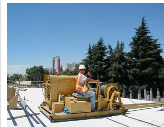
Photo 4-11 – Tendon Pulling Machine.
