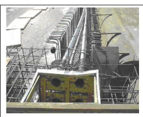
Photo 5-2 – Blockout for Anchorage Devices.
