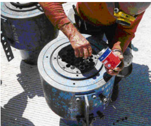
Photo 6-1 – Pulling Wedges Inserted into Jack
