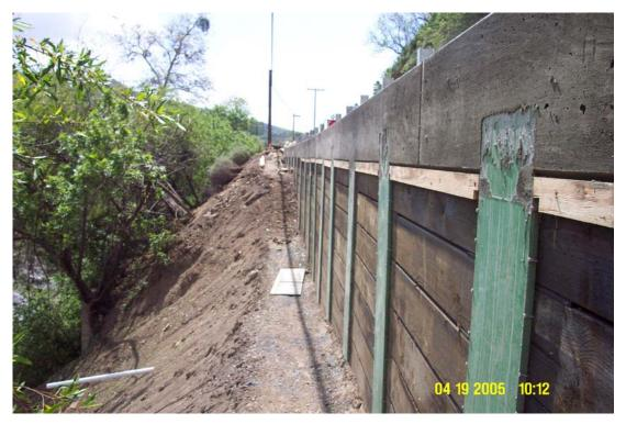
Figure 6-2. Soldier Pile Wall with Cap Beam
