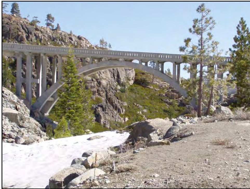
Photograph 6: Open Spandrel Arch, Donner Summit Bridge (17C0052), Nevada County. May 2003.
