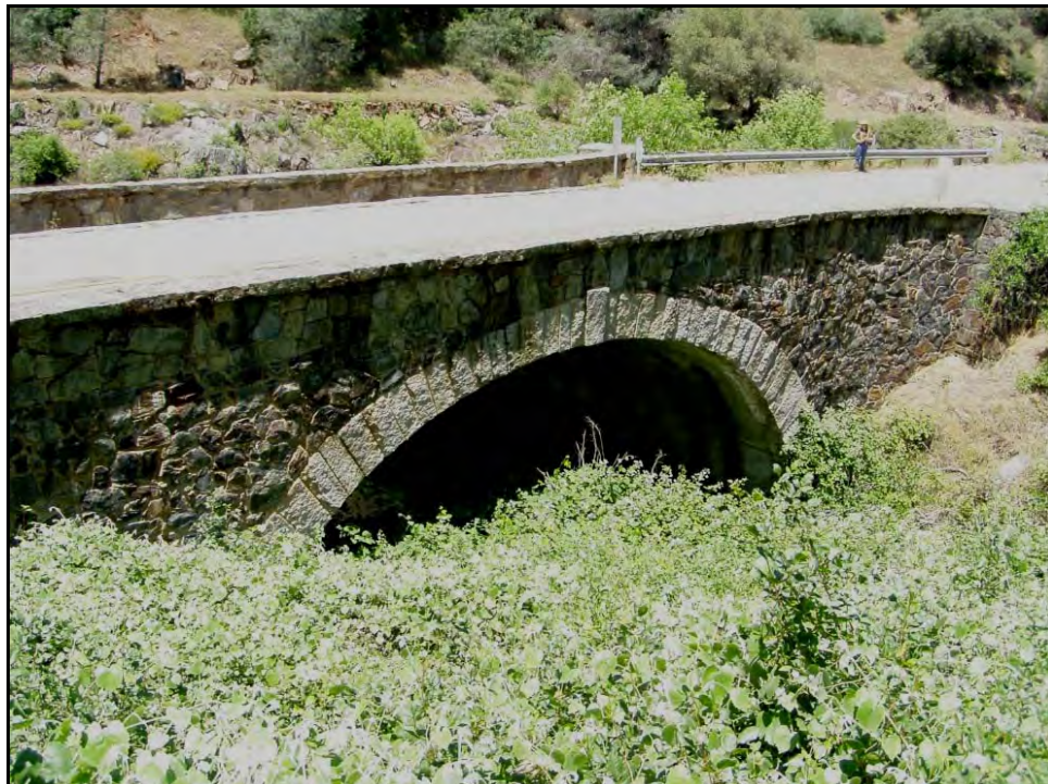
Photograph 7: Masonry faced Sweetwater Creek Bridge (40 0007) on Highway 140, Mariposa County. May 2003.
