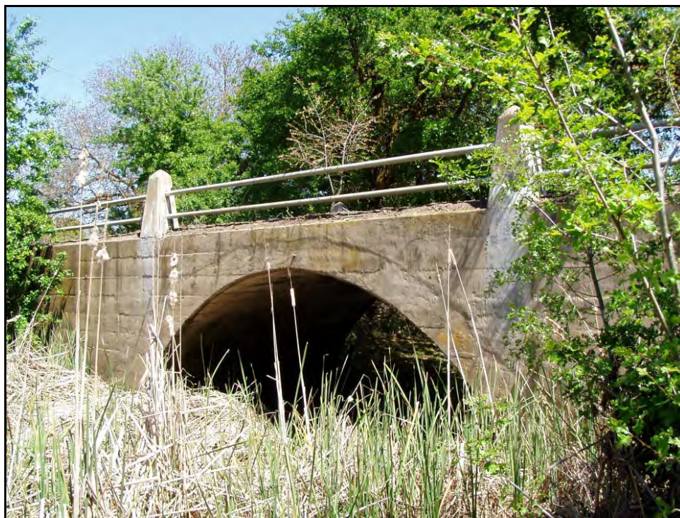
Photograph 5: Closed Spandrel Arch, Dry Slough Bridge (22C0121), Yolo County. April 2003.
