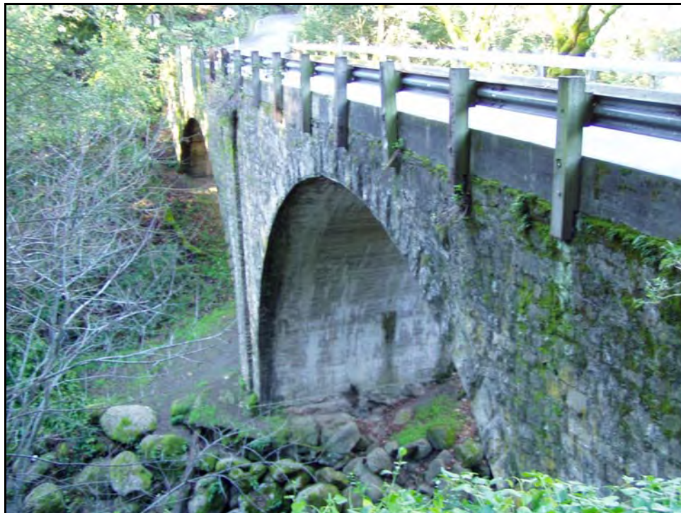
Photograph 2: Saratoga Creek Bridge (37 0074), built 1902. February 2003.
