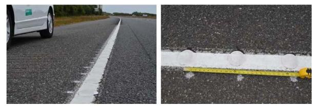
Figure 12: Photographs of Type A raised pavement markers (dots) installed on US Highway 101
