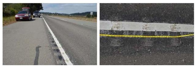
Figure 11: Photographs of ground rumble strips on State Route 299
