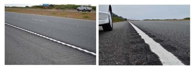
Figure 7: Photographs of mumble strips installed on US Highway 101
