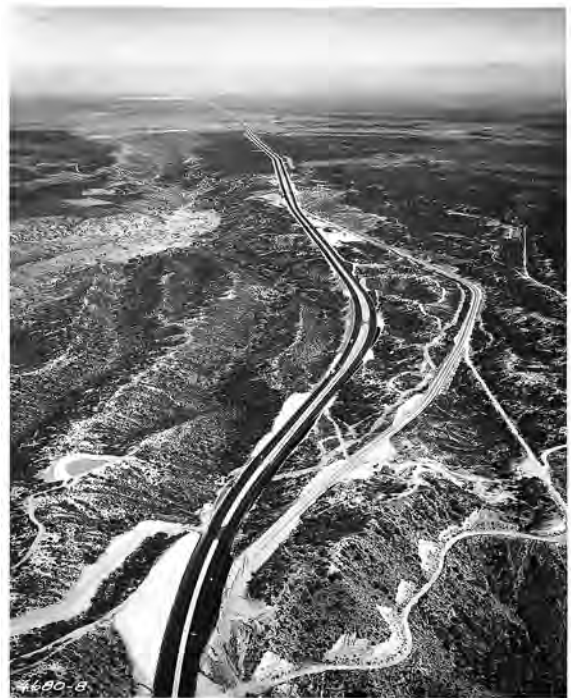
Figure 83. Route 66 improvements in Bernardino County, ca. 1960s (Caltrans Transportation Library, Sacramento).
