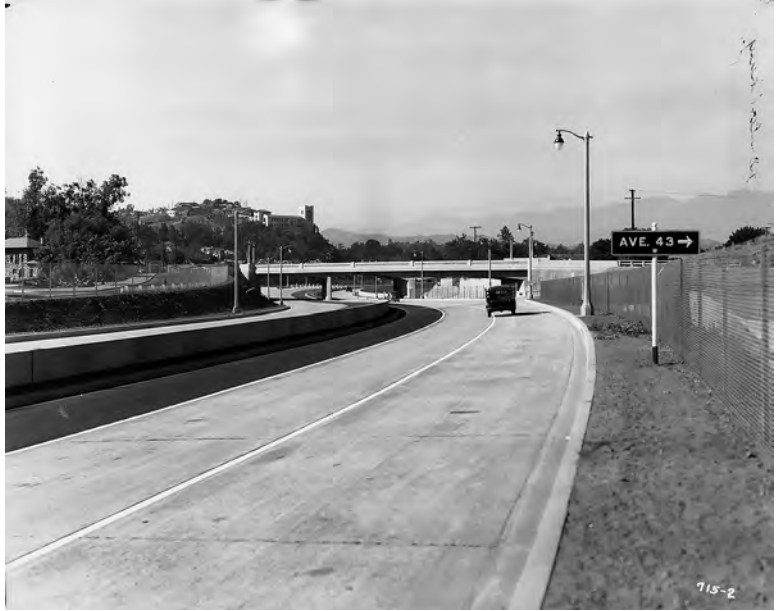
Figure 22. Arroyo Seco Freeway, July 1940. The Arroyo Seco or Pasadena Freeway was designed for both aesthetics and engineering (Caltrans Transportation Library, Sacramento).
