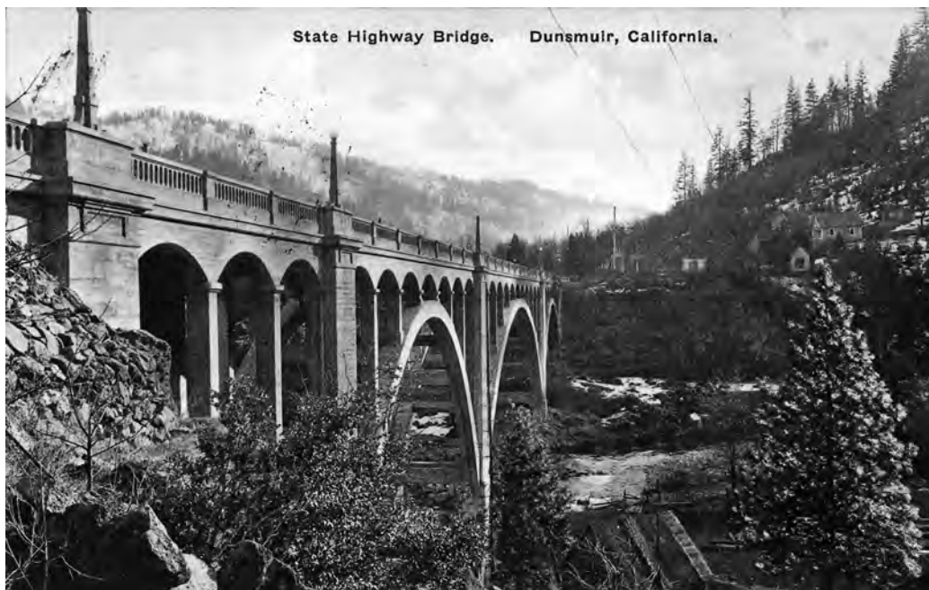
Figure 103. Dunsmuir reinforced concrete arched bridge following completion in late 1910s (Bedford Collection, Caltrans Transportation Library, Sacramento).
