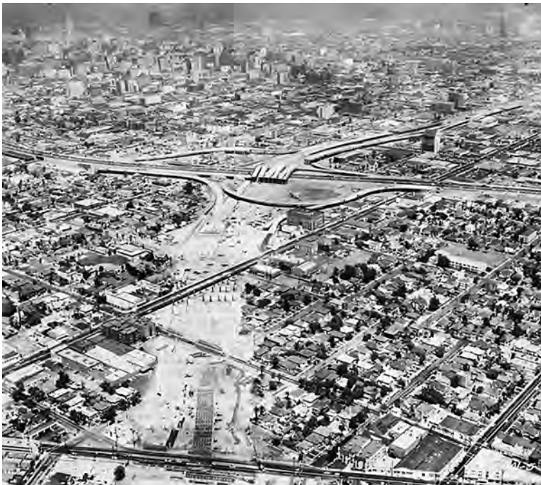
Figure 89. Construction of the Santa Monica Freeway divided neighborhoods and displaced residents. Here, work continues on the freeway southwest of downtown Los Angeles in the 1960s (California Division of Highways, Sacramento. Date: 6-22-61; neg. no: 8201-5; district: VII; county: Los Angeles; route: 173).
