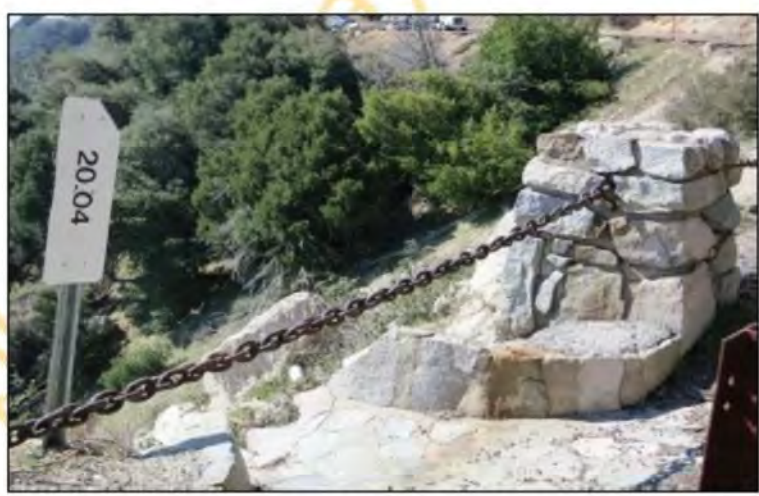
Detail of rubble masonry "pier-and-chain" guardrail, View west at P.M. 20.04.
