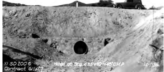
Figure 110. Typical cut-and-fill and culvert construction along San Diego 200 (SR 94), 1934. Note the concrete-masonry headwall that was common through the 1910s–1930s (Caltrans Transportation Library, Sacramento).
