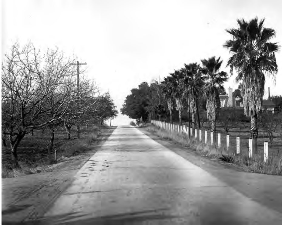
Figure 108. Concrete highway, Orangevale, Sacramento County, 1917 (Caltrans Transportation Library, Sacramento).
