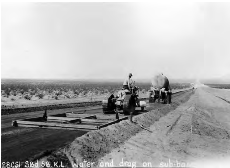
Figure 82. Route 36 under construction, San Bernardino County, ca. 1931 (Caltrans Transportation Library, Sacramento).
