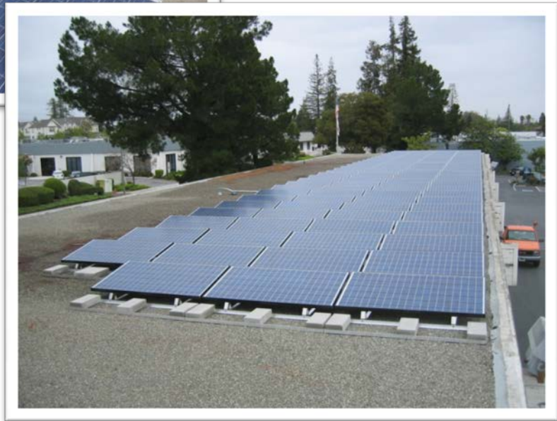
District 4 Cupertino Maintenance Station
