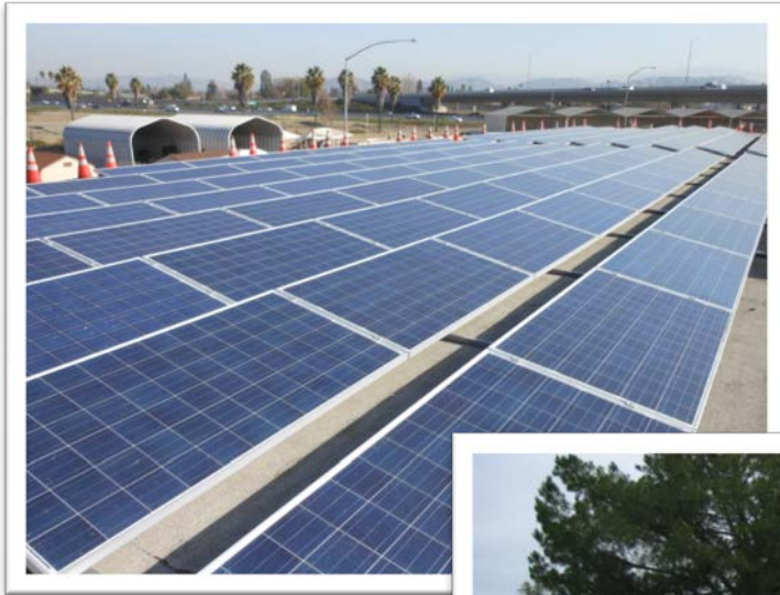
District 12 Orange Maintenance Station
